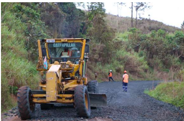
Rural road rehabilitation works in Natua Labasa.
