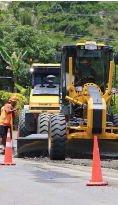
Road work on Hibiscus Highway, near Savusavu Airport.
