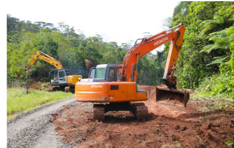
Drainage works on a section of rural road in Vanua Levu.
