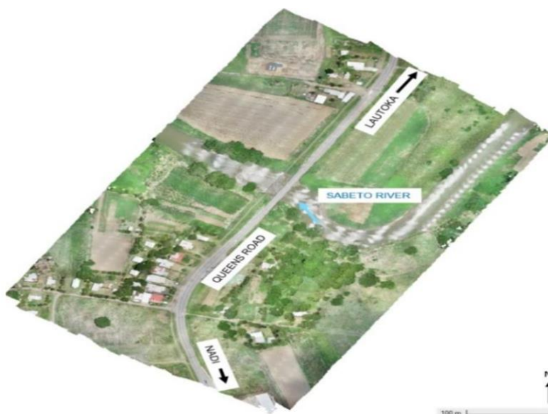
Figure 1.9: Sabeto Bridge aerial
