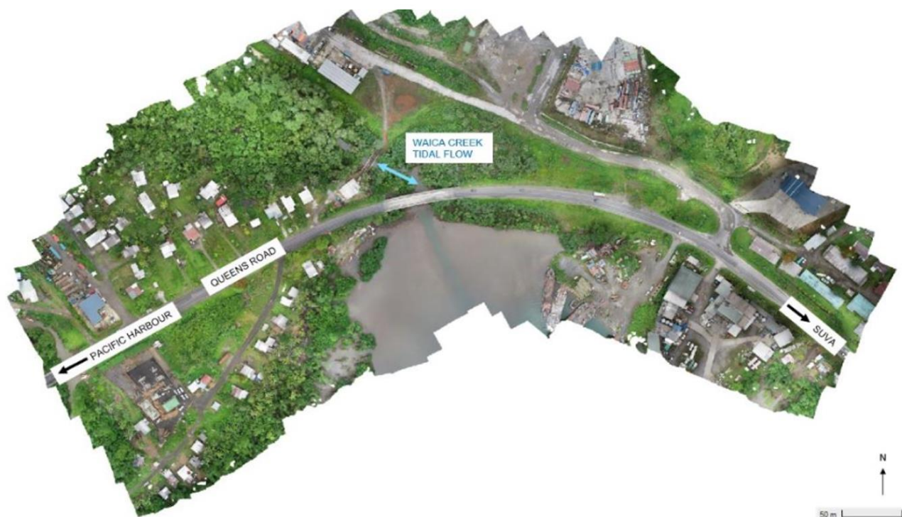
Figure 1.7: Medraukutu Bridge aerial
