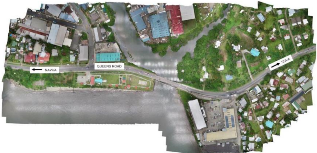
Figure 1.9: Lami Bridge aerial
