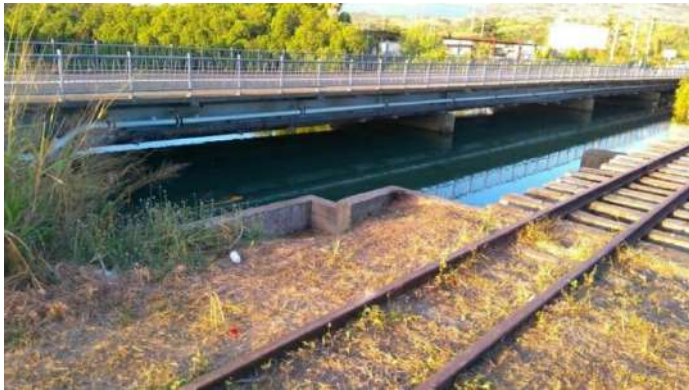
From downstream elevation (FRA, 2016)
