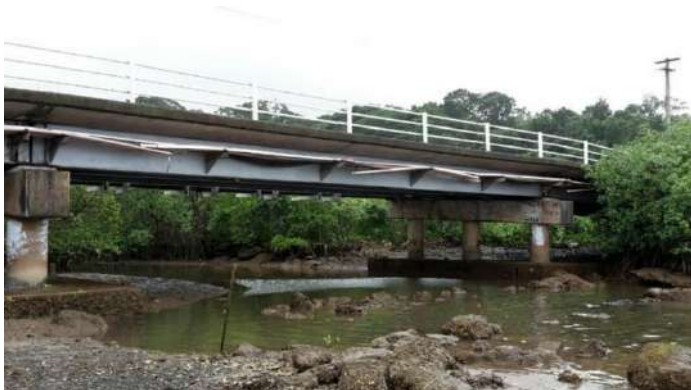
From downstream elevation (FRA, 2016)
