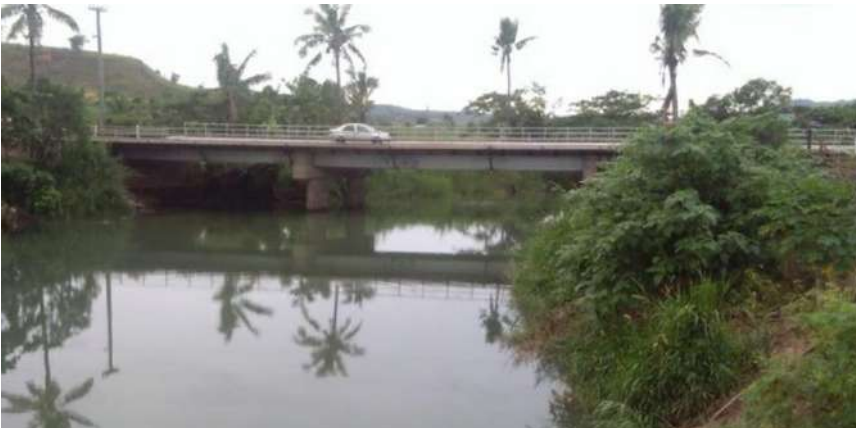
From downstream elevation (FRA, 2016)
