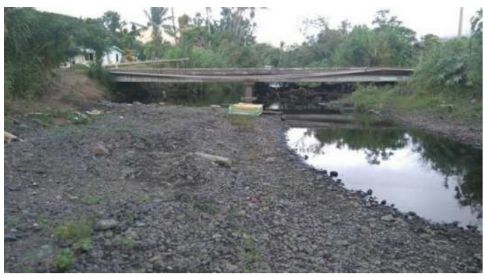
From downstream elevation (FRA, 2016)
