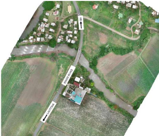
Matawalu bridge aerial
