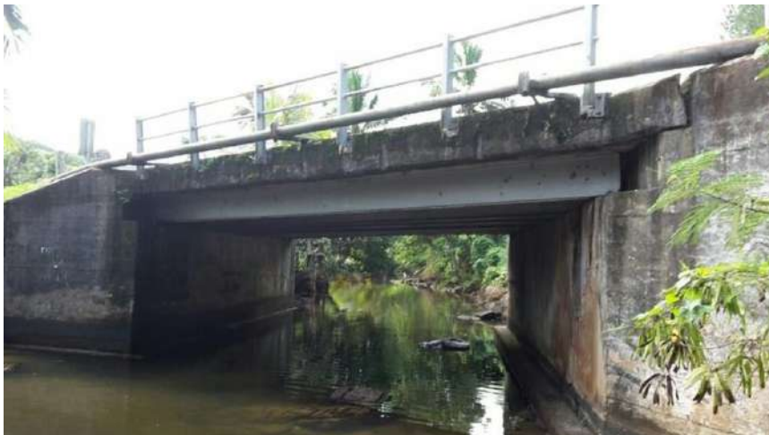
From downstream elevation (FRA, 2016)
