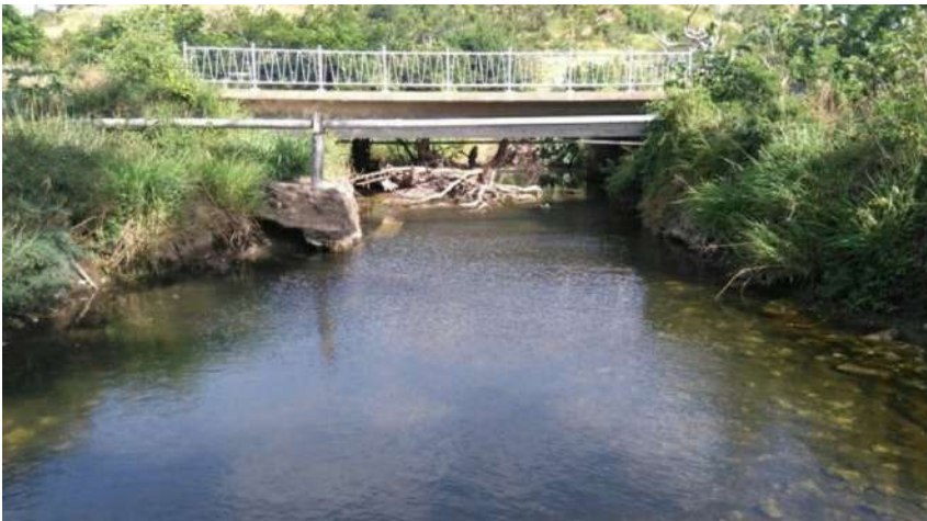
From downstream elevation (FRA, 2016)
