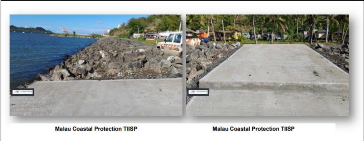
Figure 7 – Malau Coastal Protection, Northern Division
