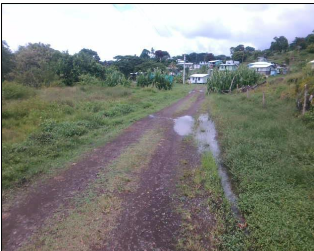
Figure 6 – Saioko Village Road, Western Division
