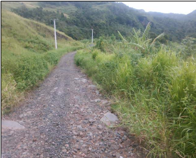
Figure 5 – Nakorotubu Road, Western Division
