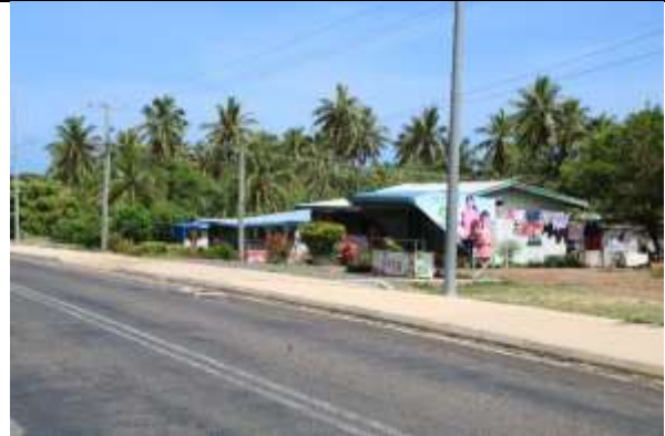
Figure 10: Newly improved footpath adjacent to existing road side stalls.
