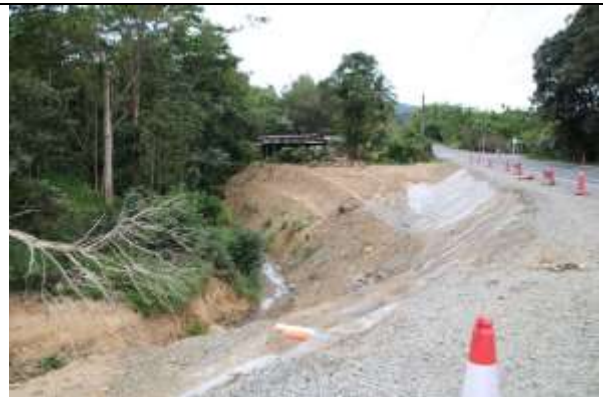
Figure 6: Slope Protection work at Navutu Section.
