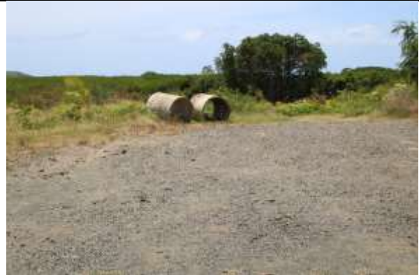
Figure 16: Culverts at a decommissioned site.
