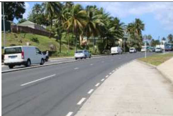
Figure 3: New improved road at Foster Road.
