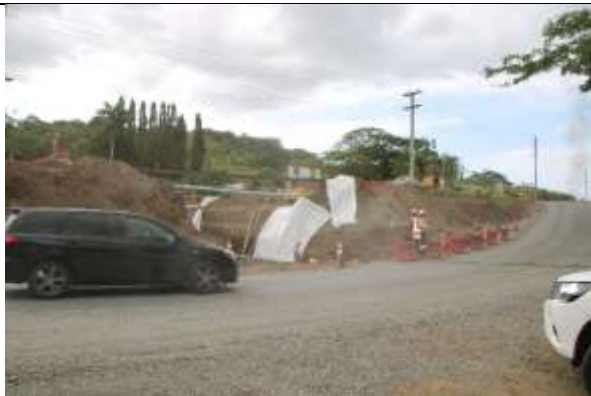
Figure 7: Culvert replacement work at Navo Section.
