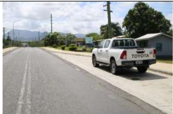
Figure 12: Improved footpath and bus-bay.
