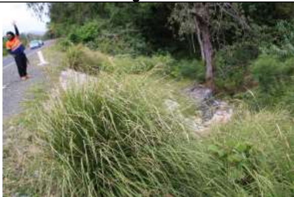
Figure 5: Vetiver Grass for slope protection.
