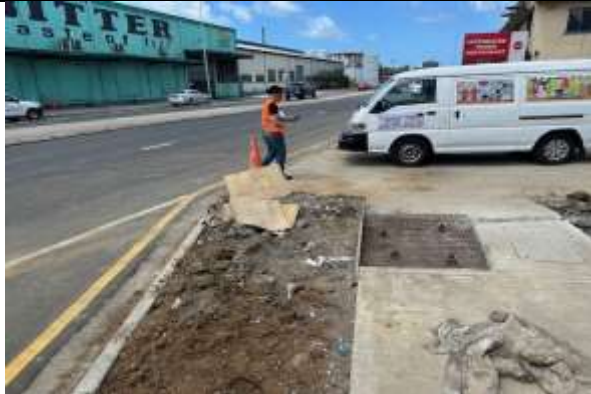
Figure 1: Foster Road Project road pavement works.
