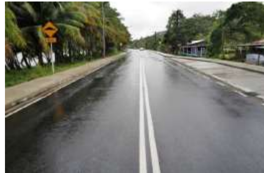
Image 4: Namada Village after upgrade works.
