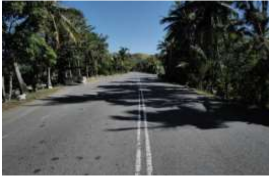
Image 1: Korotogo Village before upgrade works.
