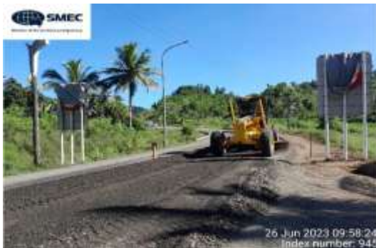
Image 5: Overlaying works along Kings Road.
