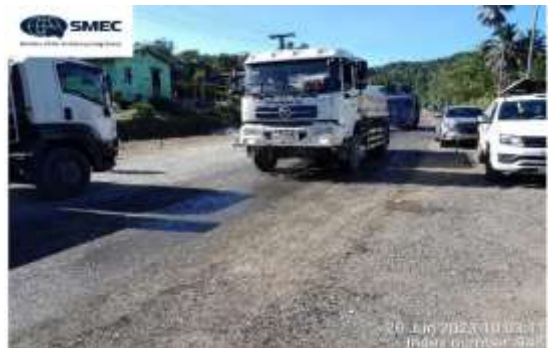
Image 6: Water cart on site to suppress dust.
