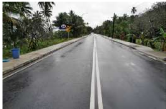
Image 6: Namada Village Suva approach before upgrade works.
