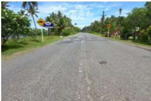
Image 5: Namada Village Suva approach before upgrade works.
