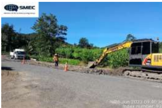
Image 3: Existing seal removal.
