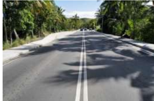
Image 2: Korotogo Village after upgrade works.
