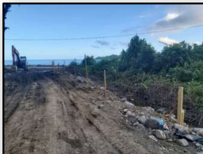
Photo 1: Nukutocia Quarry Fencing and Rehabilitation works.
