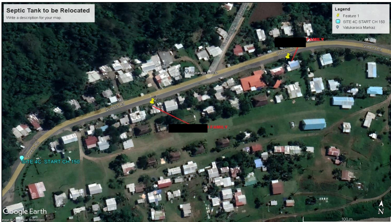
Figure 1 – Locality of the 2 Affected Houses
