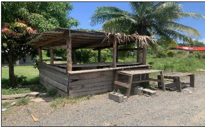
Temporary Wooden Stall used occasionally by villagers. Outside Road Reserve.
