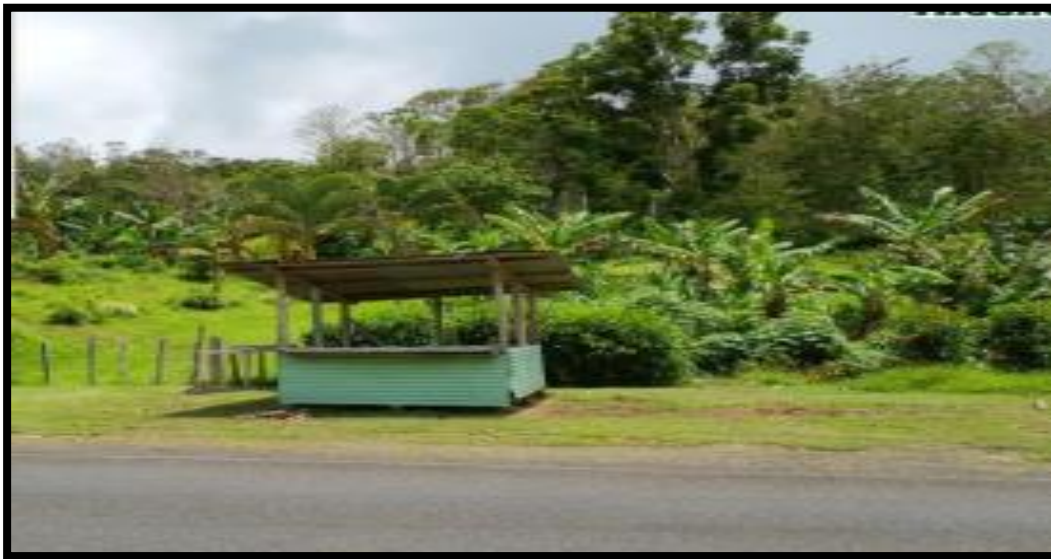
Figure 2 –Corrugated Iron Roofing Stall
