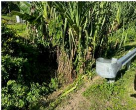
Figure 4: Guardrails relocated further in land.
