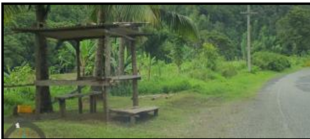
Figure 4 – Stall of Corrugated Iron Roofing with 4 wooden posts
