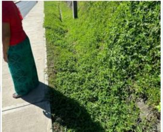
Figure 5: Overgrown drain
