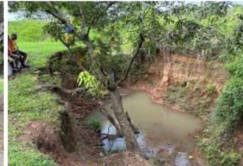
Figure 9: Continuous scouring leading to loss of land.
