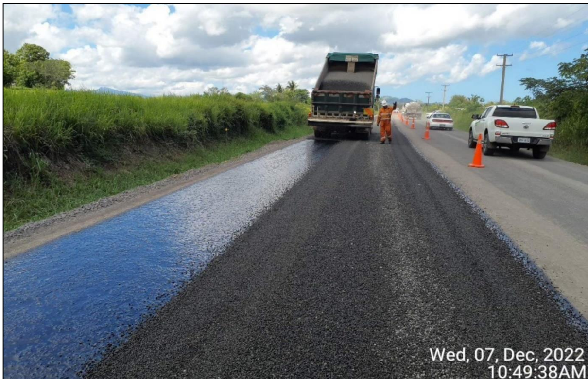
Figure 17 – Shows ongoing constructions and traffic management plan
