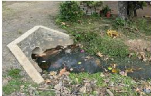
Figure 7: Blackwater discharge from residence to the new drainage system,
