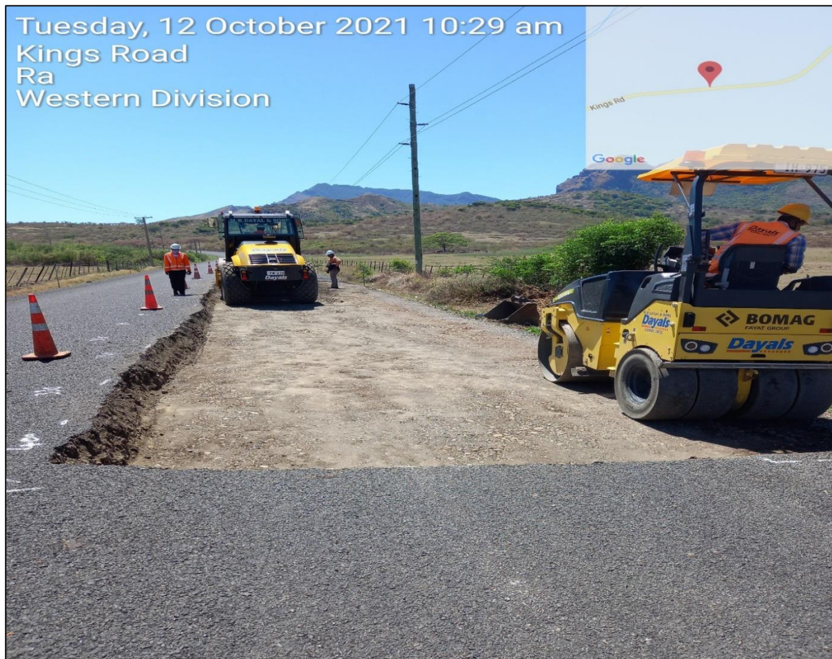
Figure 18 – Shows ongoing constructions
