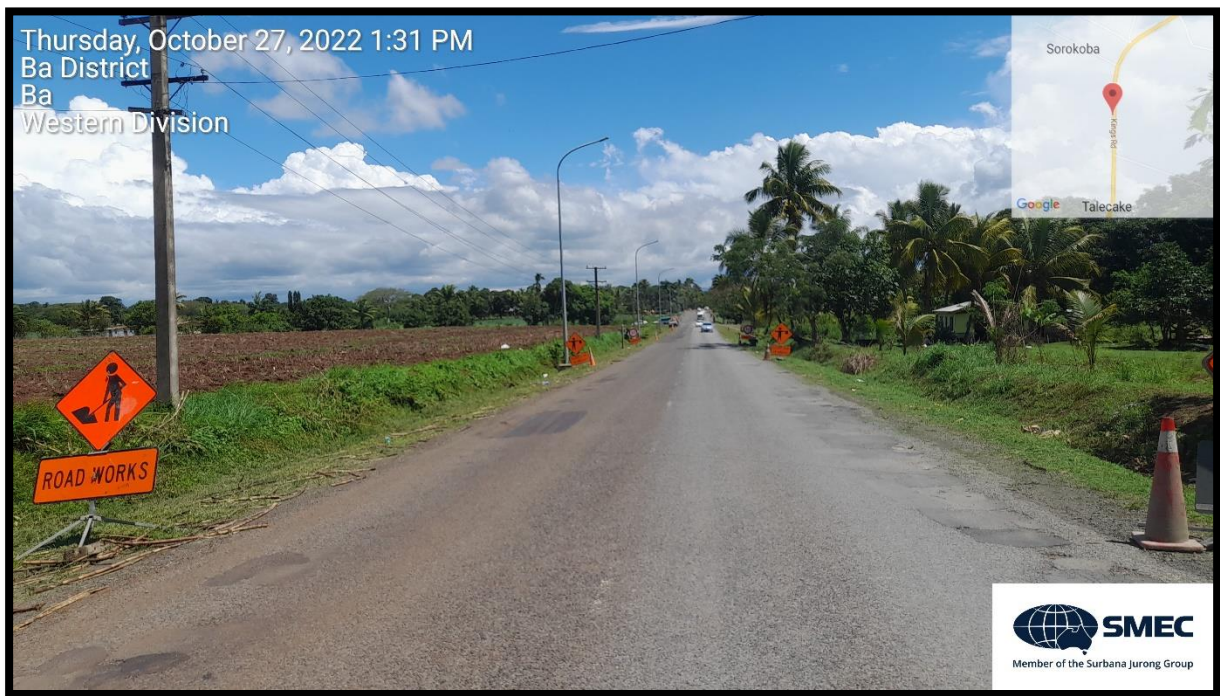
View of Road Stretch from Sorokoba Village
