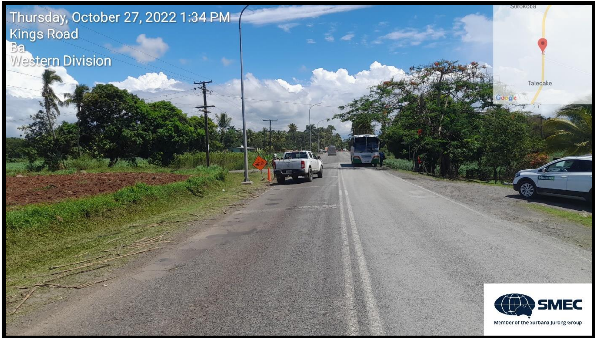
View of Access Roads on both sides towards Natalecake Village. Contractors will provide a TMP to manage the continued and safe access.
