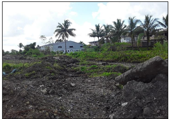
Unlevelled surface of the Subject Area
