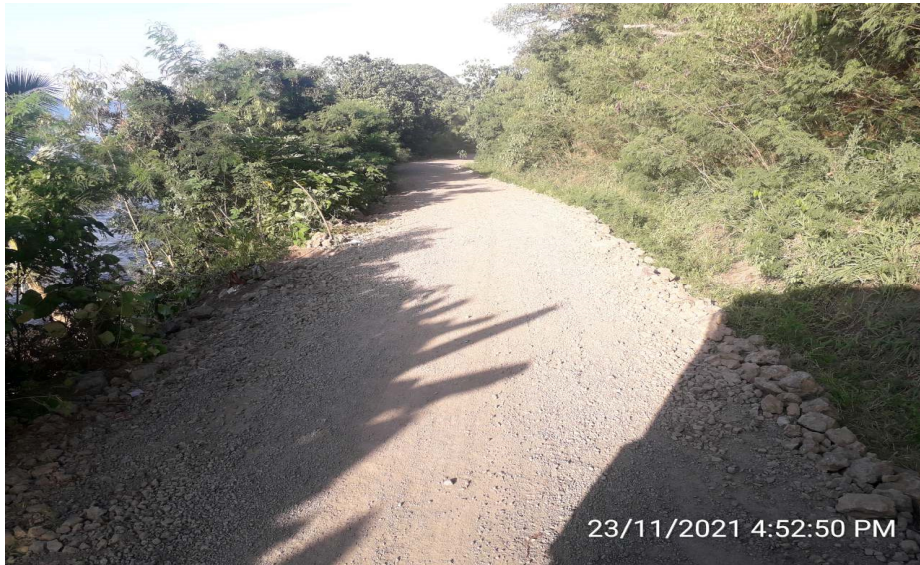
Partly Section of Rabi Coastal Road where the incident occurred
