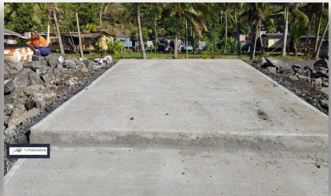
Malau Coastal Protection TIISP
