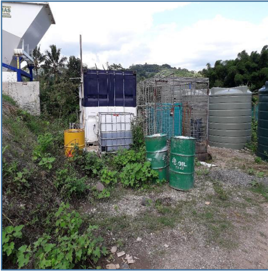
Photo 1 – Oil drums not enclosed in bunded area
