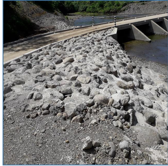
Photo 2 – Crossing abutment rip-rap
