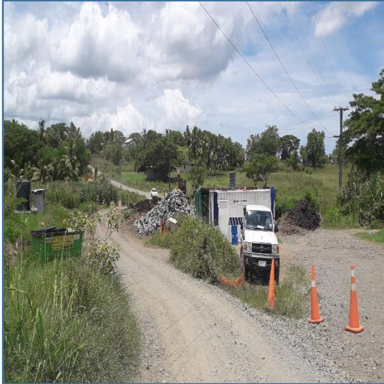
Photo 1 – Project Laydown Area
