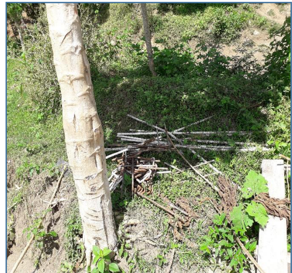
Photo 4 – PVC pipes and iron rods dumped carelessly on site.
