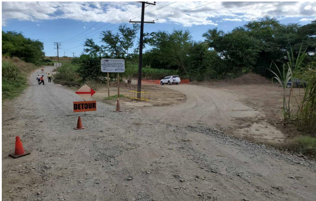
Photo 8: Site office access, detour and installed GRM signboard.
