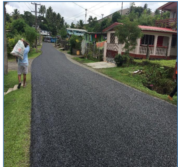
Photo 4 – Completed Resal Site.
