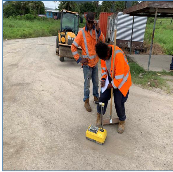
Photo 2 – Quality assurance checks along Queen’s Road.
