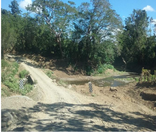
Figure 1: Site prior to re-construction.
