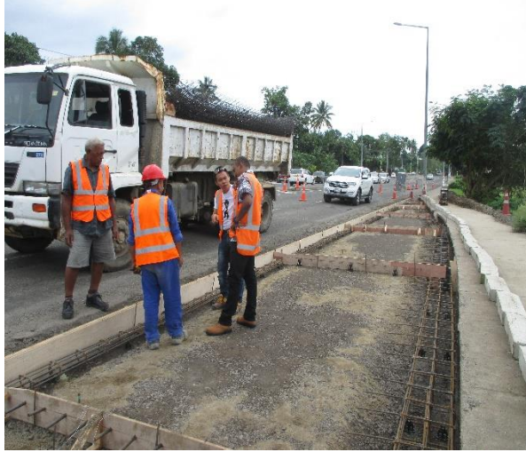
Figure 1: Onsite discussion between FRA Senior Engineer and Contractors
