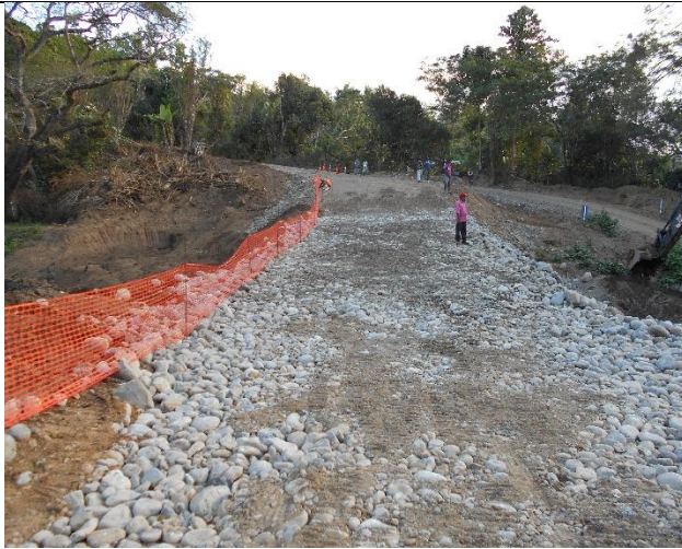
Figure 3: Temporary crossing diversion located upstream.
