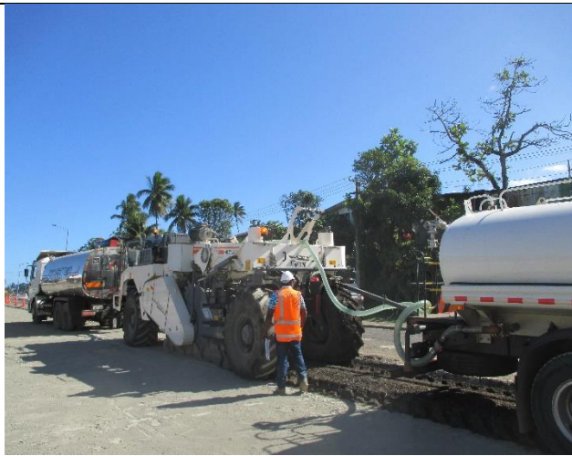
Figure 3: FBS process being supervised by FRA Engineer.
