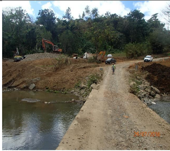
Figure 4: Mobilization onto site.
