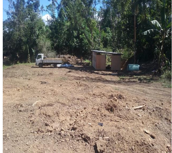
Figure 2: Temporary site yard preparation by Contractors.
