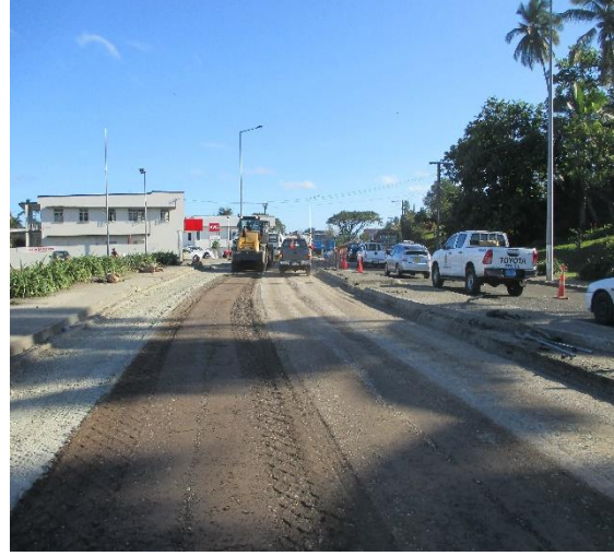
Figure 2: Foam Bitumen Stabilization (FBS) in process.
