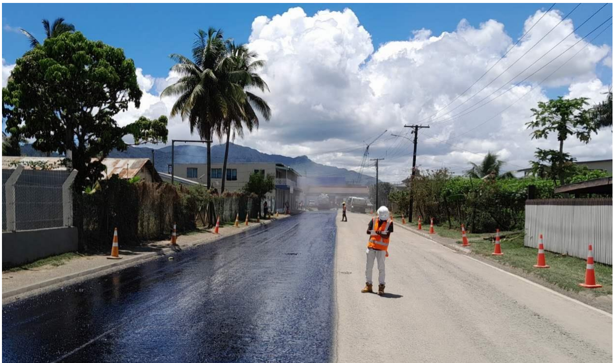
Sealing in progress at Silas Ramzan Street, Labasa.
