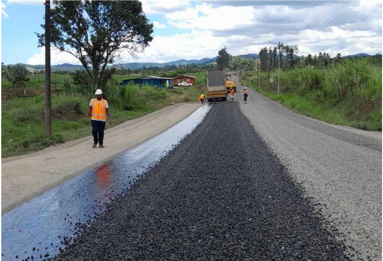
Road works progressing on Navidamu Road.
