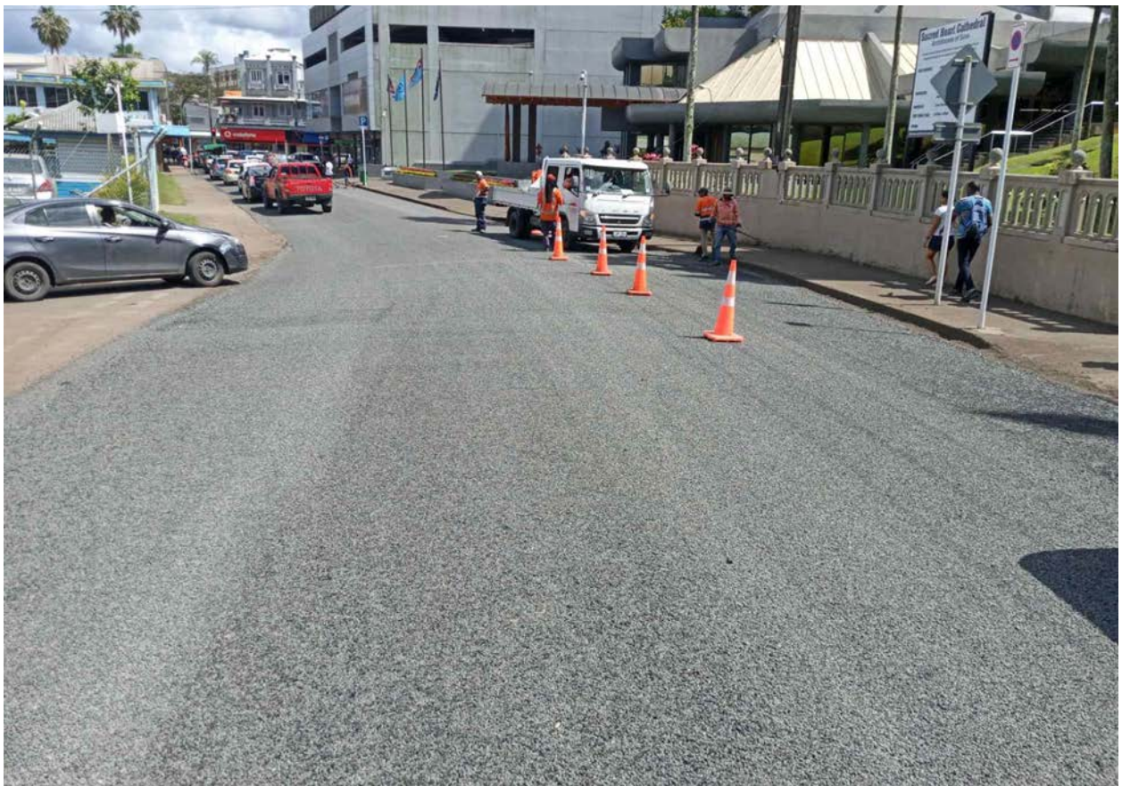
Resurfacing works on Pratt Street, Suva under Pot Hole Preventative Maintenance Program
