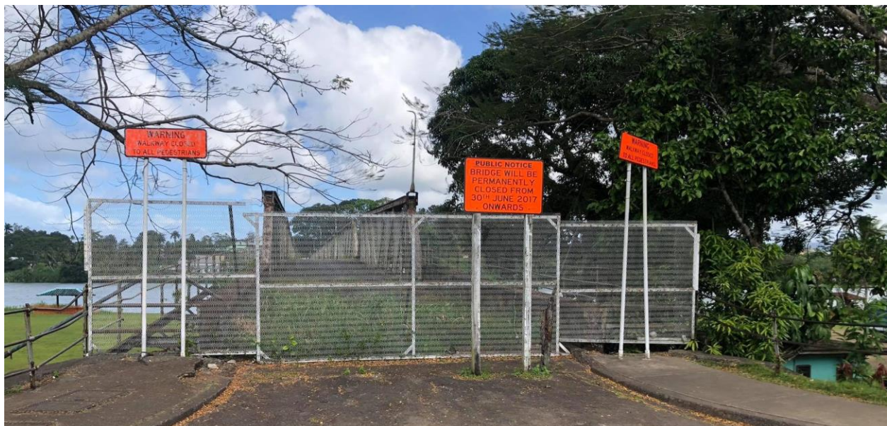
The old Rewa Bridge was closed indefinitely for public safety.
