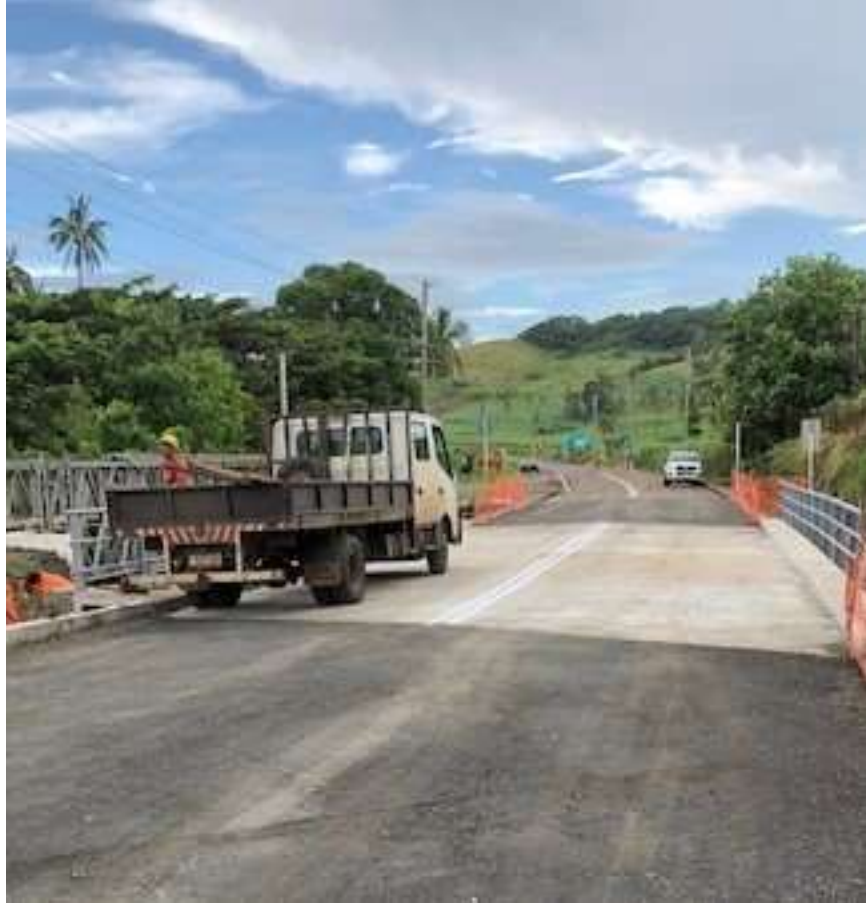
New and improved Vatudova Bridge
