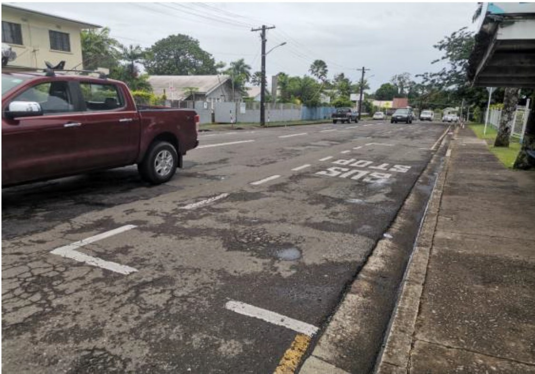
MacGregor Road in Suva to undergo rehabilitation works from tonight
