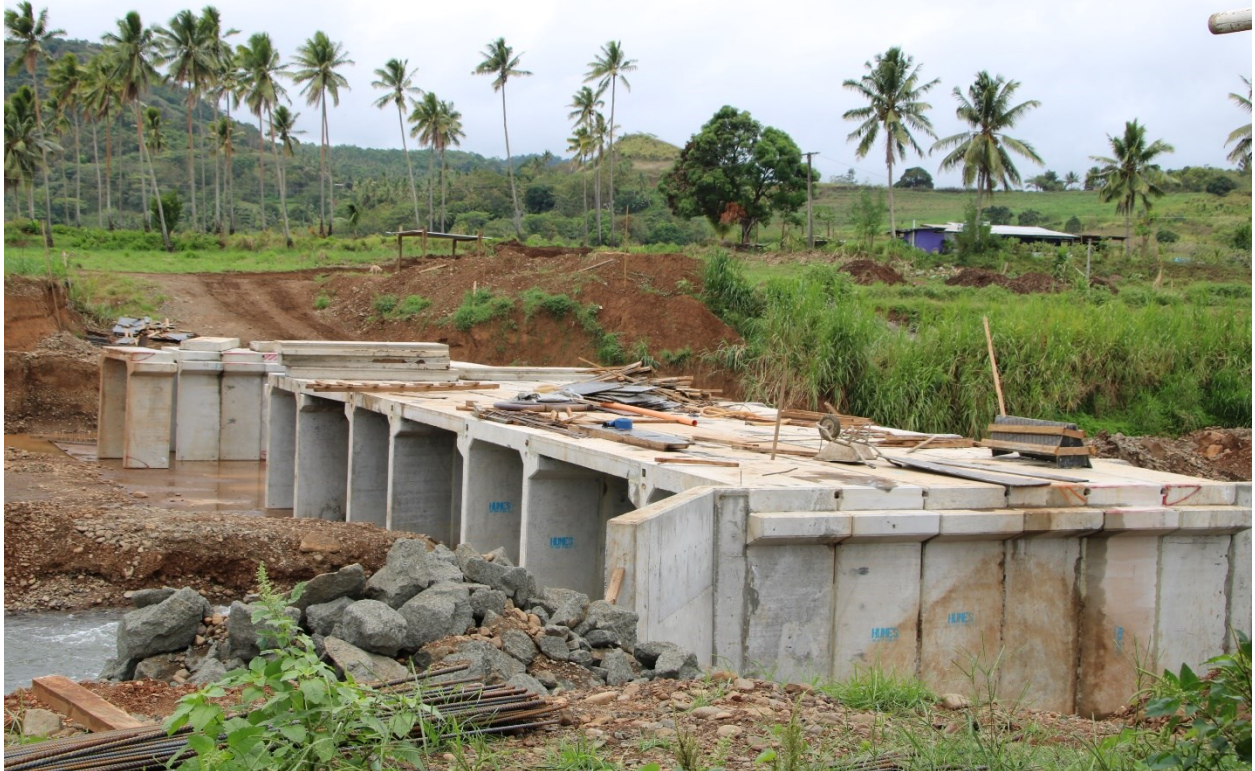
Works on Nakorotari Crossing progressing well
