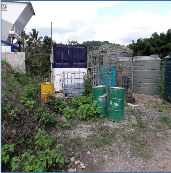
Photo 1 – Oil drums not enclosed in bunded area
