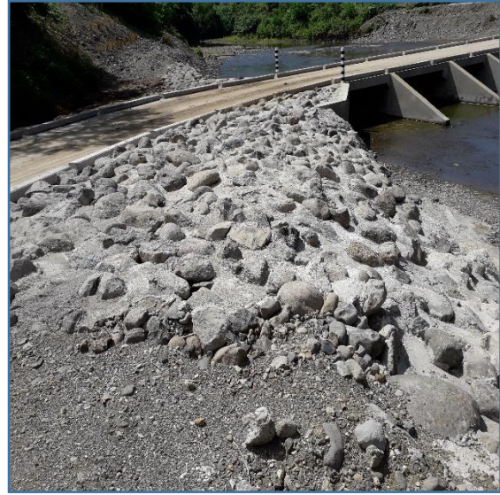
Photo 2 – Crossing abutment rip-rap
