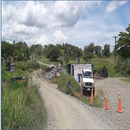
Photo 1 – Project Laydown Area
