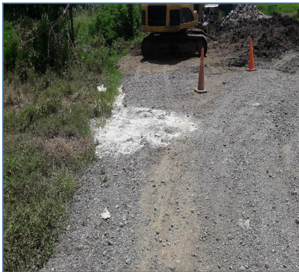
Photo 3 – Spilled cement on the road.
