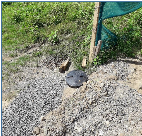
Photo 3 – Portable septic tank still installed and has not been removed off site.
