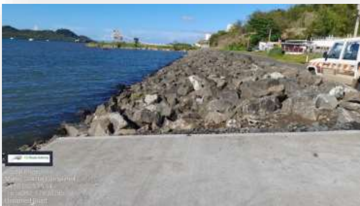
Malau Coastal Protection TIISP
