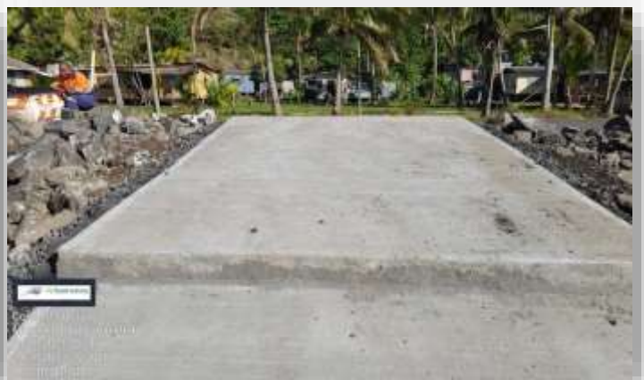
Malau Coastal Protection TIISP
