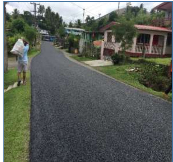
Photo 4 – Completed Reseal Site.
