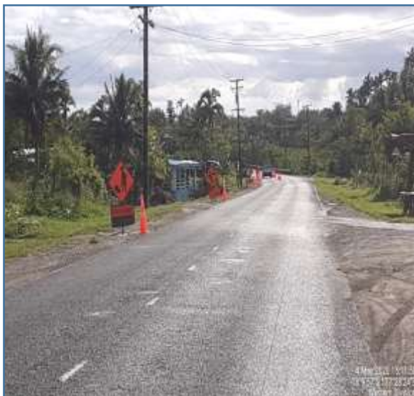
Photo 3 – High shoulder removal works
