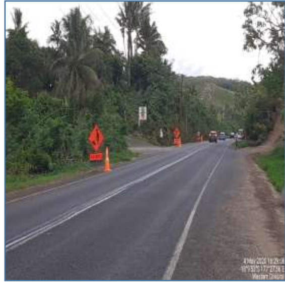
Photo 2 – High shoulder removal works
