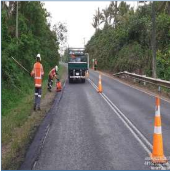
Photo 1 – Road shoulder repair works
