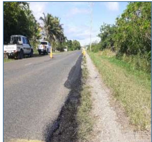
Photo 4 – Road shoulder repair works
