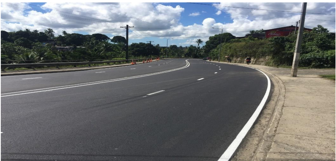
Rehabilitation work on Ratu Mara Road
