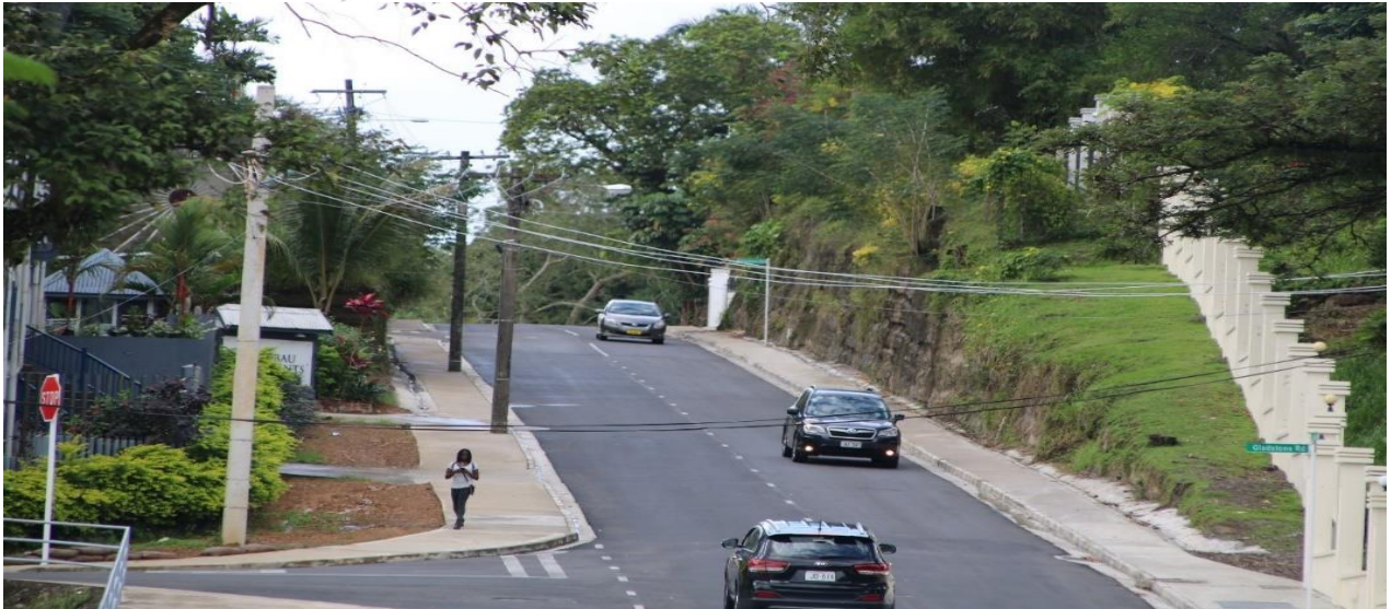
Rehabilitation works completed at Ratu Cakobau Road in Suva
