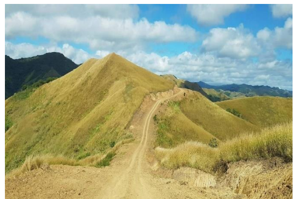
Works in progress at Matokana Village Access Road
