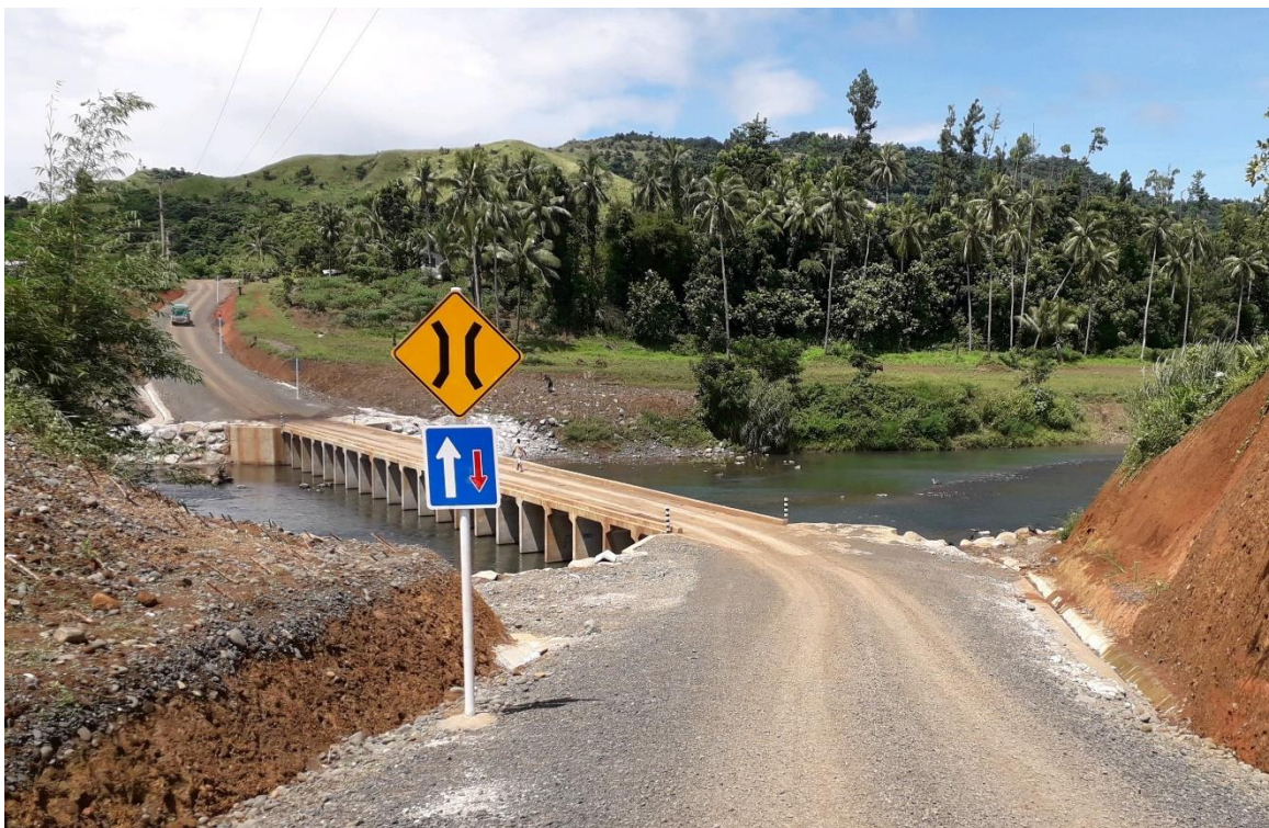
Completed works on Burelevu crossing
