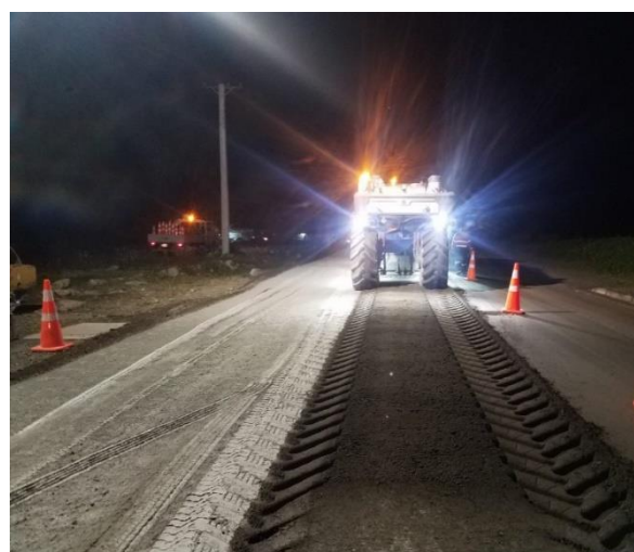
Rehabilitation works on Ratu Dovi Road
