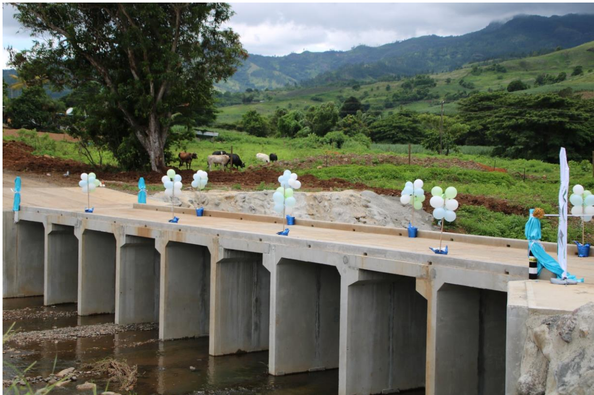
32mtr crossing providing a safe route to the residence of Vakabuli Paipai who experience regular flooding.
