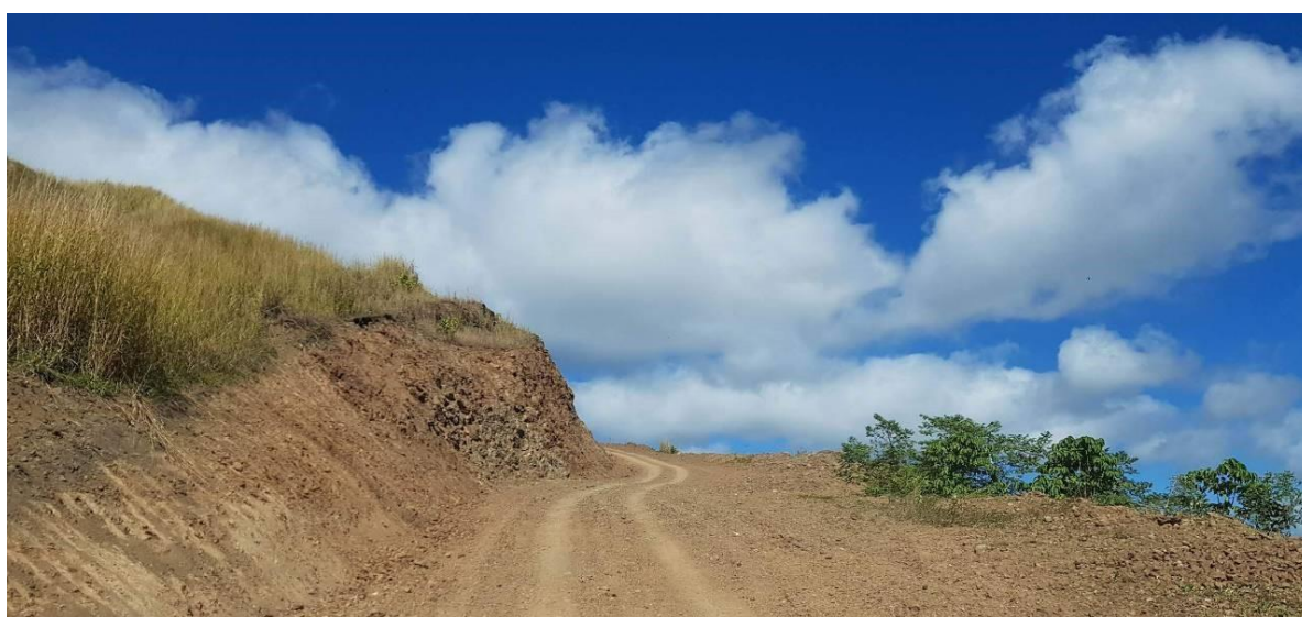
Works in progress at Matokana Village Access Road
