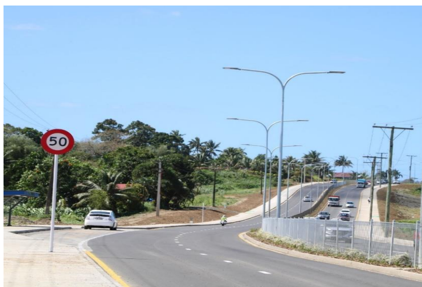
Stage 3- 4 lane road project on Kings Road between Rewa Bridge and 9-Miles.
