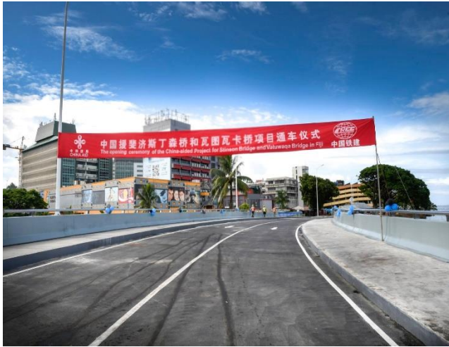
Completion of the Stinson Parade bridge in Suva.
