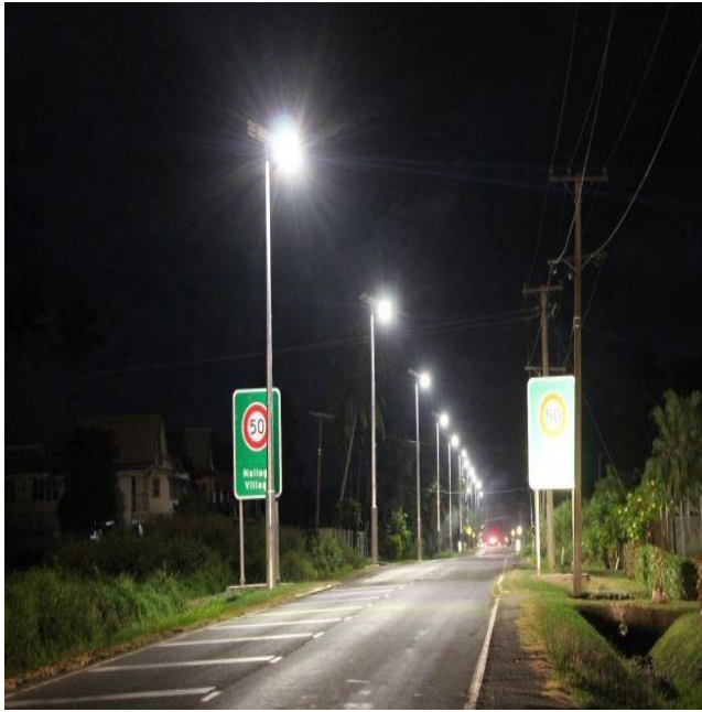
FRA's first Solar Streetlight Project in Nailaga Village in Ba.
