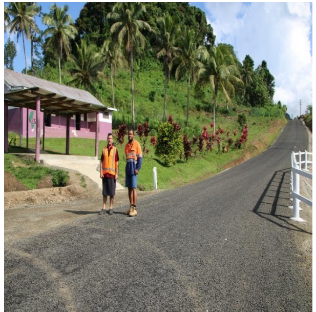
New sealed road through Naivurevure village.
