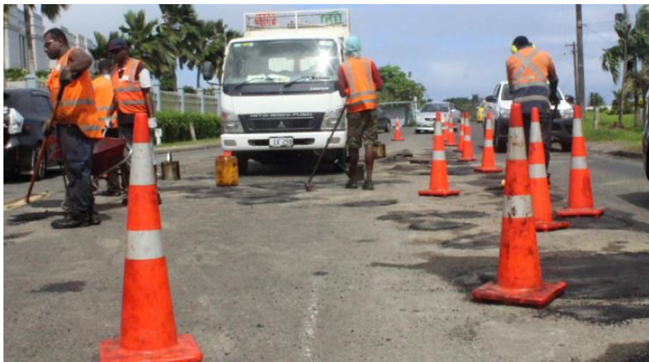
FRA works on road renewals and maintenance
