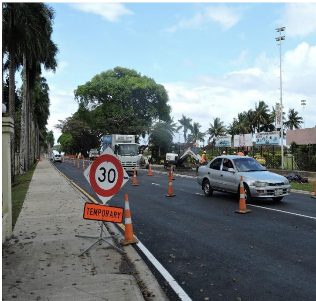
Queen Elizabeth drive road currently under work in progress.
