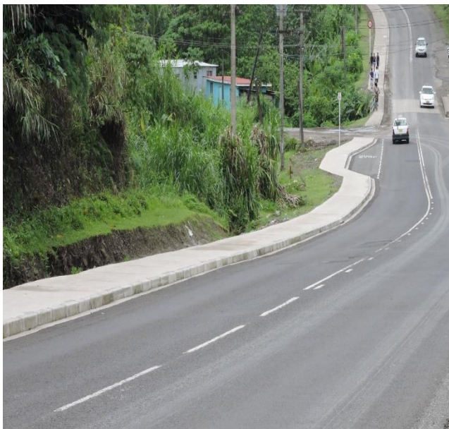
Construction of footpath along Cunningham to improve pedestrian access and safety.
