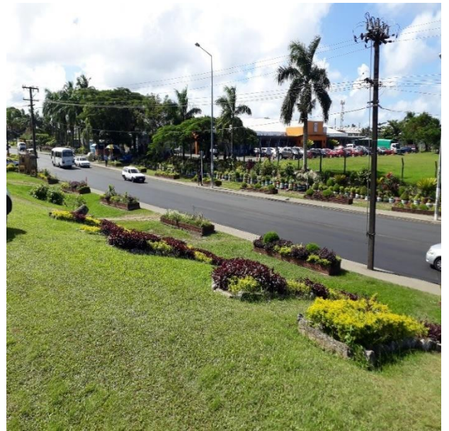
The newly upgraded Daniva Road in Valelevu, Nasinu.
