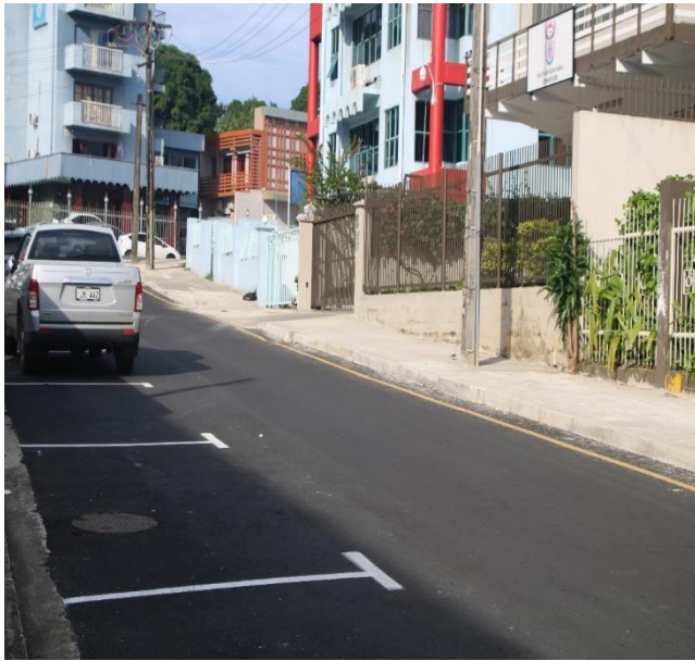
Completed rehabilitation road work at Kimberly Street in Suva.
