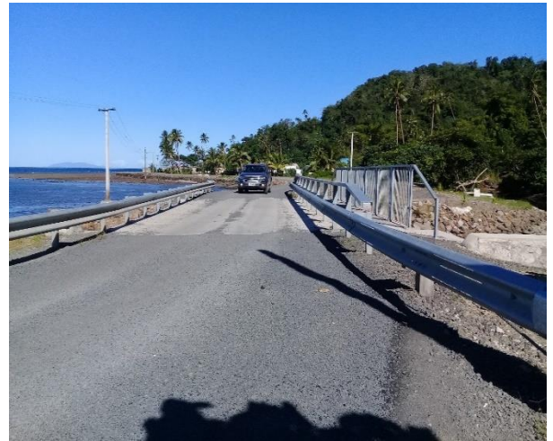
Completed construction of the Naisogo bridge in Levuka.
