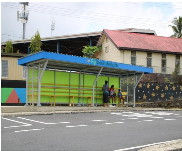
Construction of new bus shelters as part of new capital programmes.
