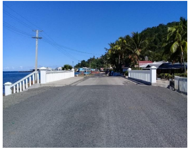
Newly constructed Levuka Market bridge.
