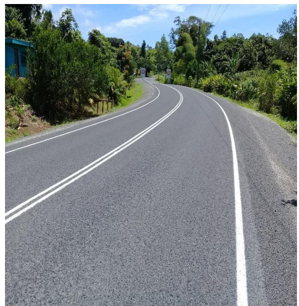
Rehabilitation works on the Naimasimasi Section on Kings Road
