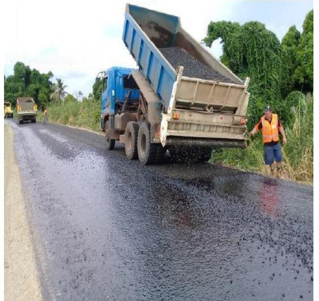
Nabouwalu to Solevu Hill traction sealing successfully completed.
