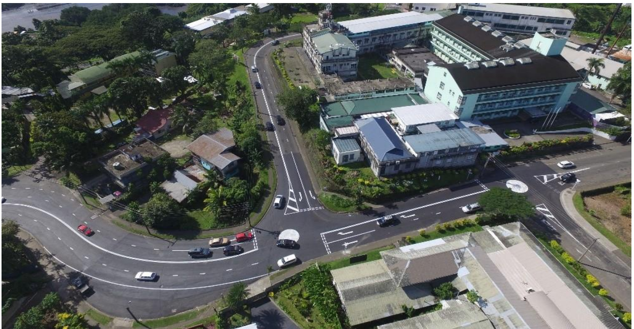
Waimanu-Brown and Brown-Amy Street roundabouts and new lane markings.
