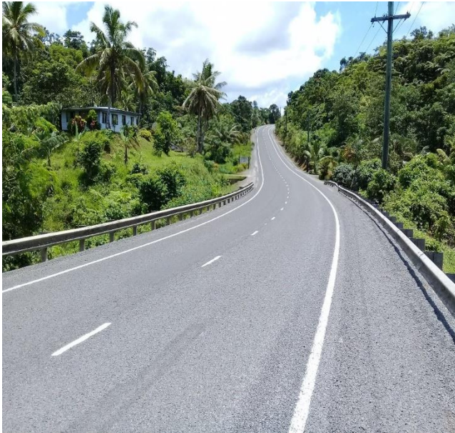
Completed rehabilitation works on the Waidalice section on Kings Road.
