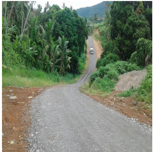
Successful completion of the new road in Moala.
