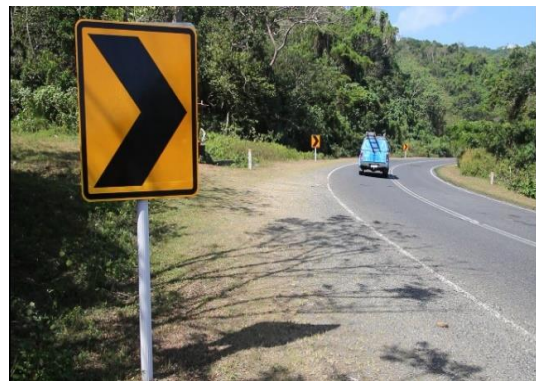
Road signs in relation to FRA's initiative in improving road safety and reducing casualties.
