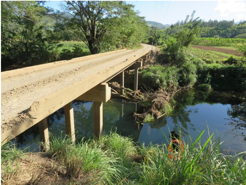
Plate 1: Narata Bridge looking west. Note the narrow width, damaged kerb, scour of abutments and accumulation of logs and debris from floods.
