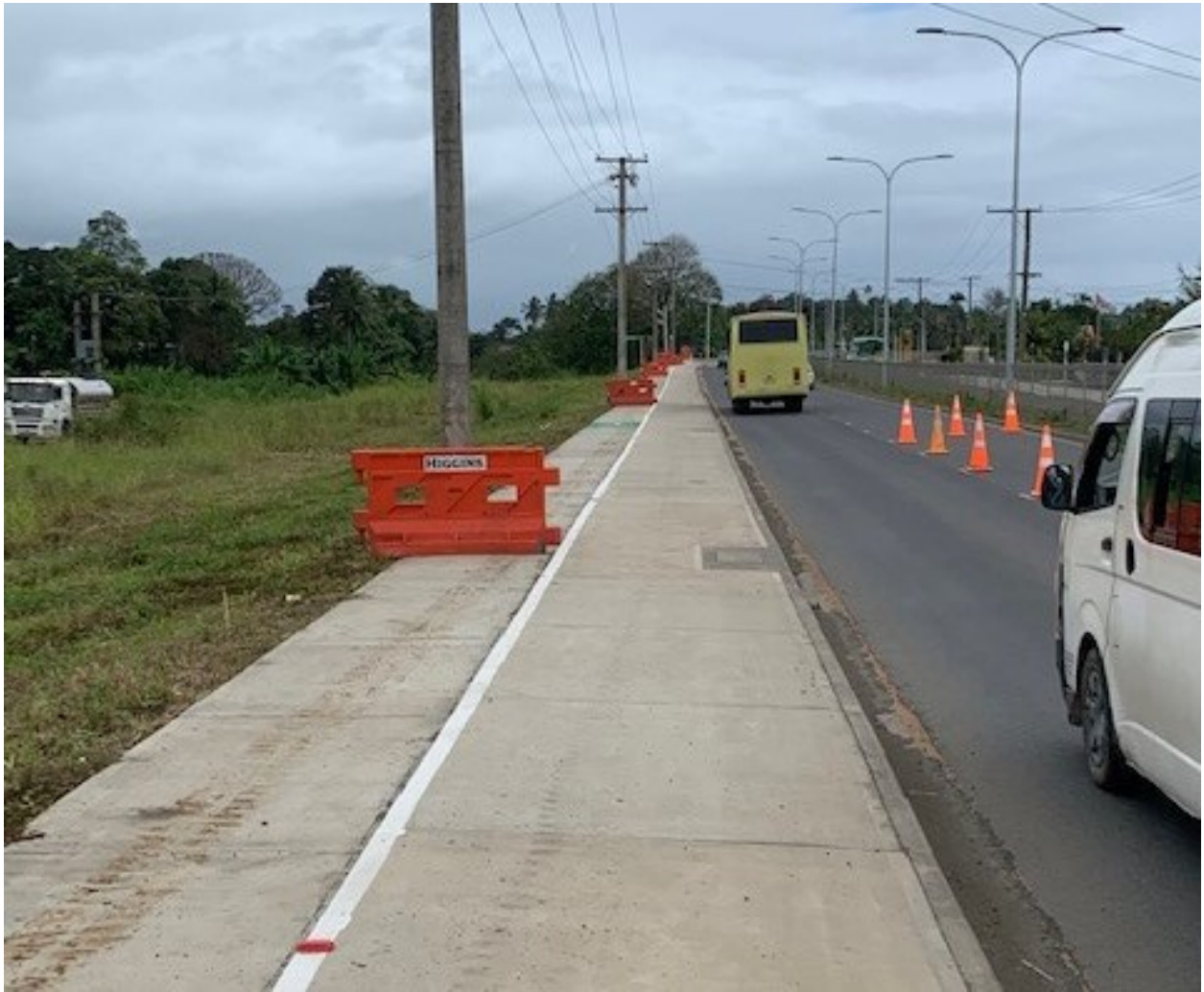
Certain sections of the cycle lane has been closed with barricades.
