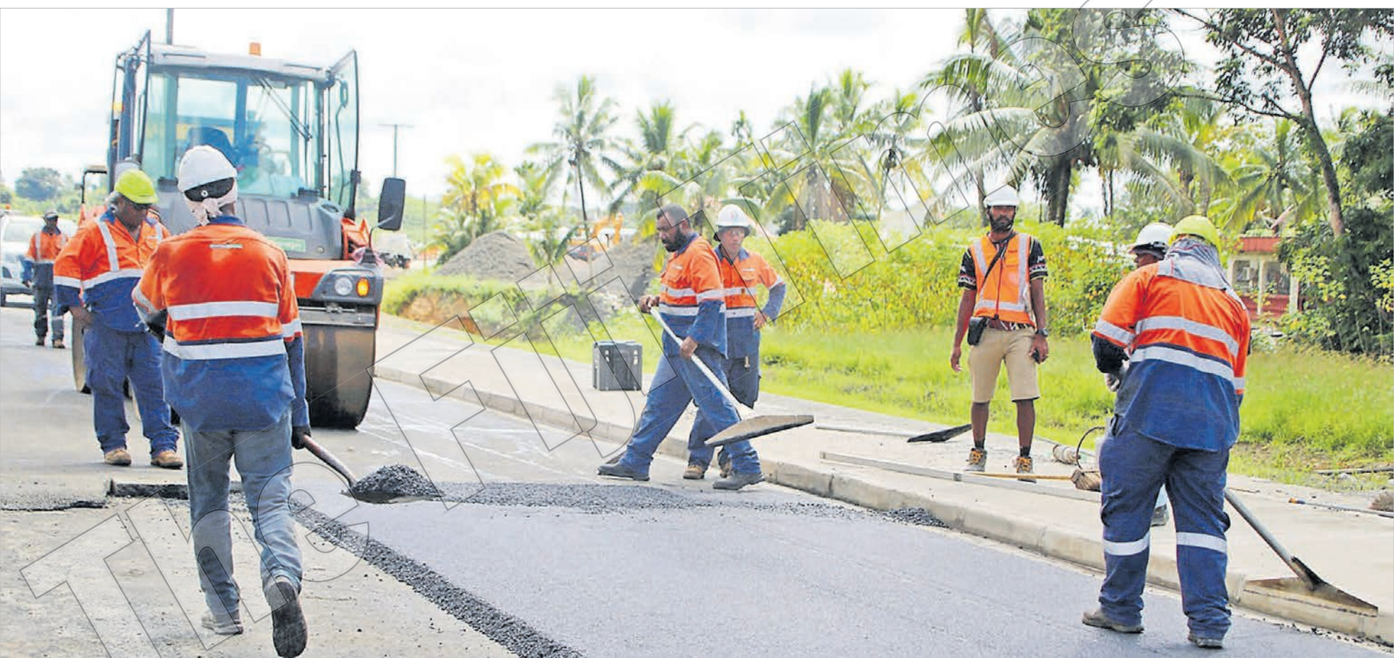
The four-lane project improves safety for all road users and greatly helps residents in their daily commuting. Picture: SUPPLIED
