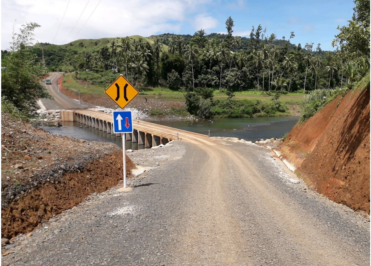
The new and improved Burelevu Crossing in Ra
