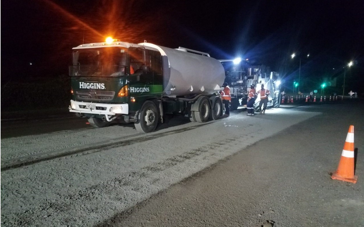
Picture Caption: Road works on Ratu Dovi Road last night.
