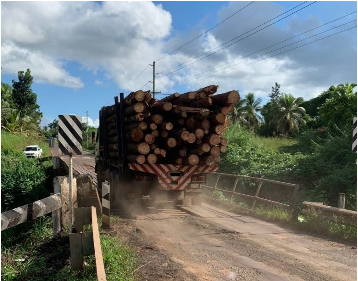
Photo Caption: An overloaded truck- a threat to road safety near the Navesidrua Village in Seaqaqa
