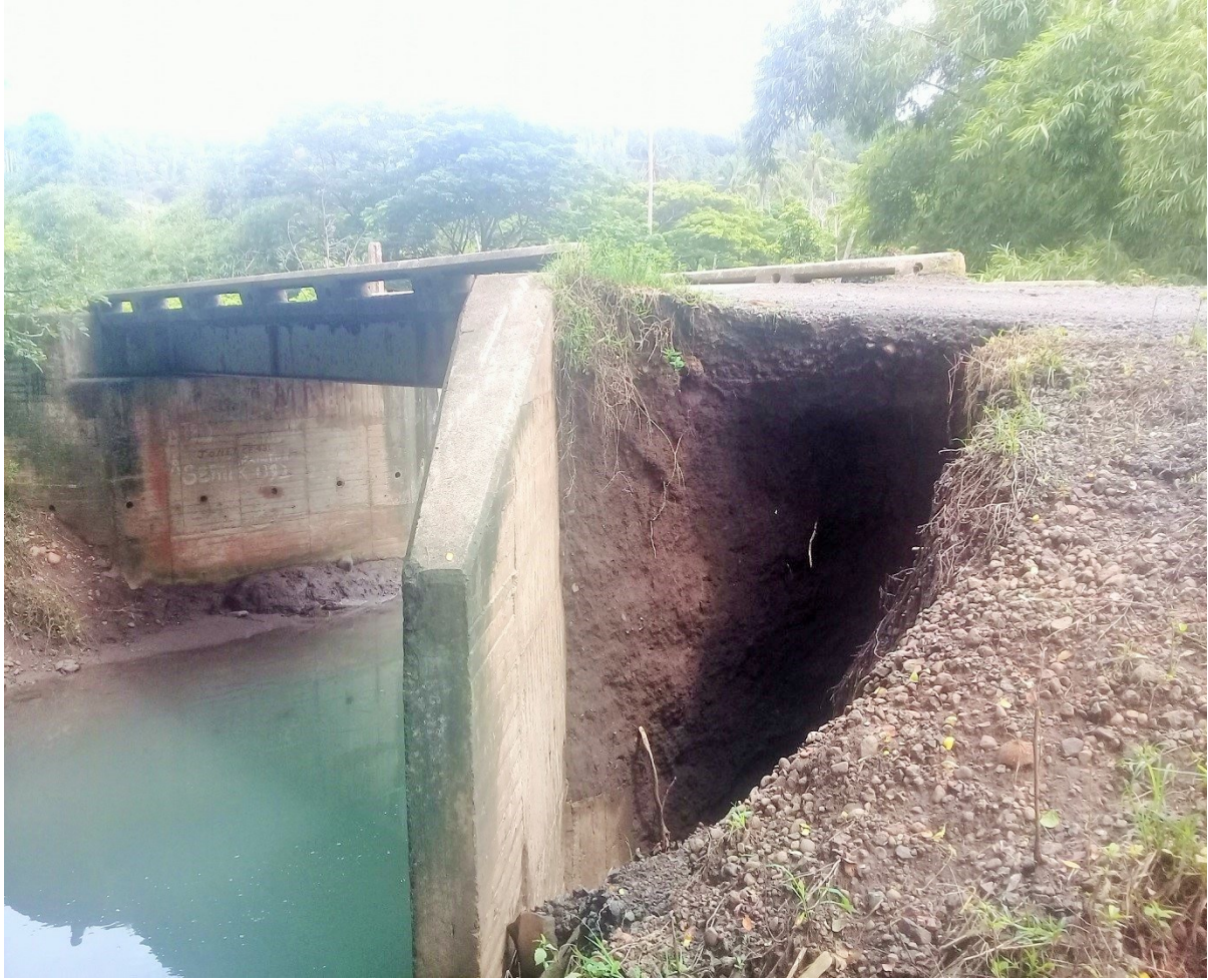
Picture Caption: Navave Crossing Approach Washout
