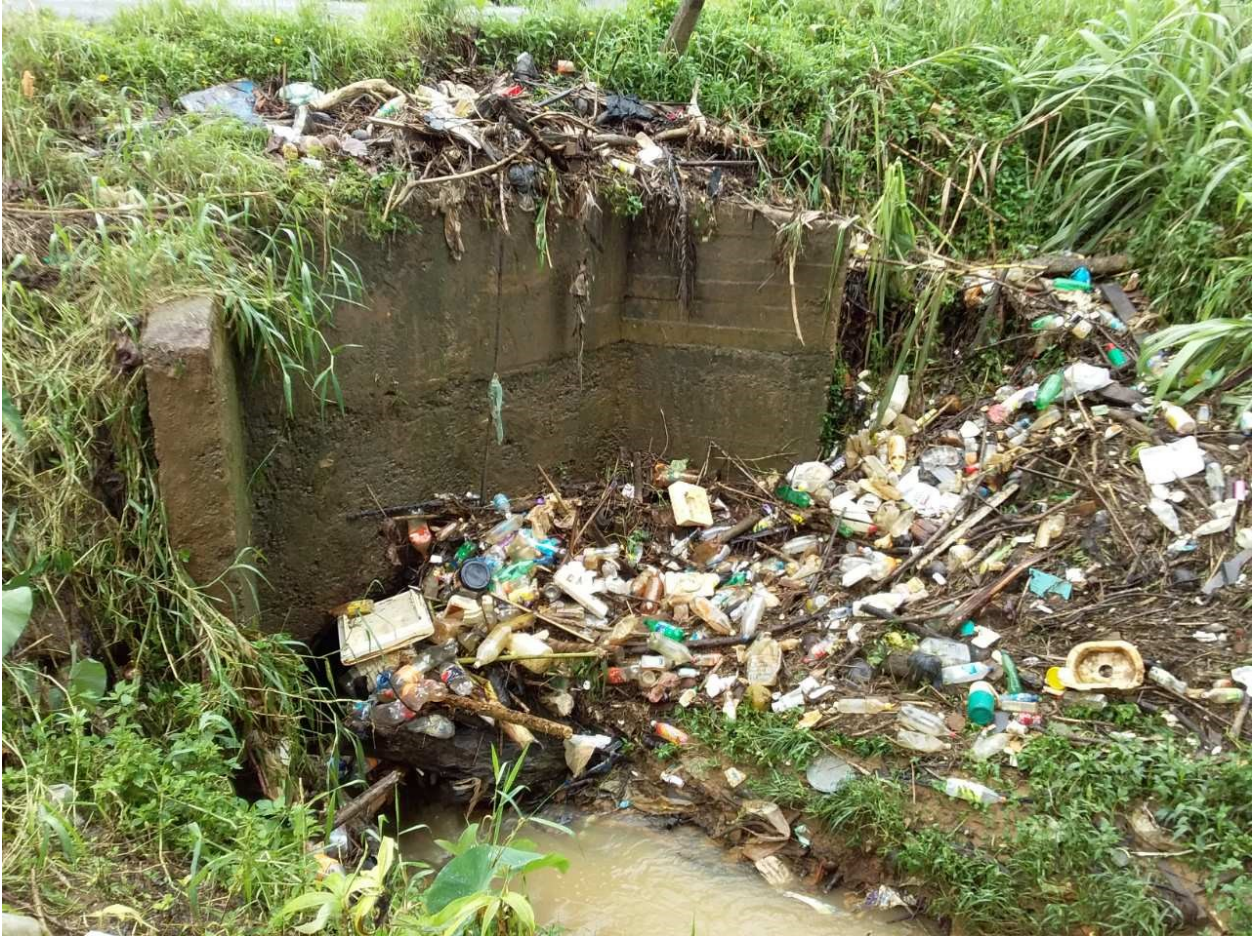
Before: The culvert crossing inlet filled with debris at Nakorovou Street in Wainibuku
