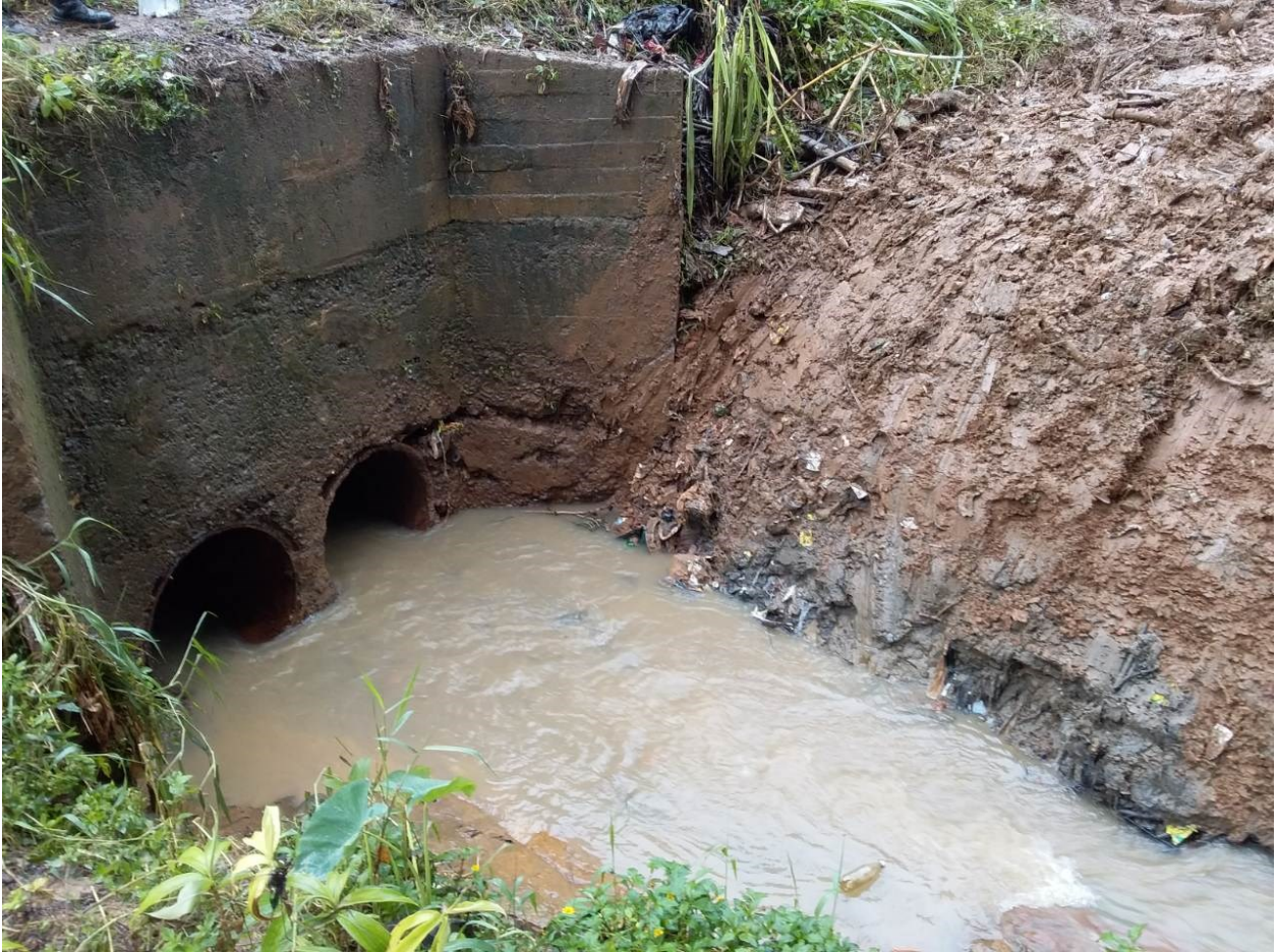
After: Debris cleared from the culvert crossing inlet at Nakorovou Street in Wainibuku
