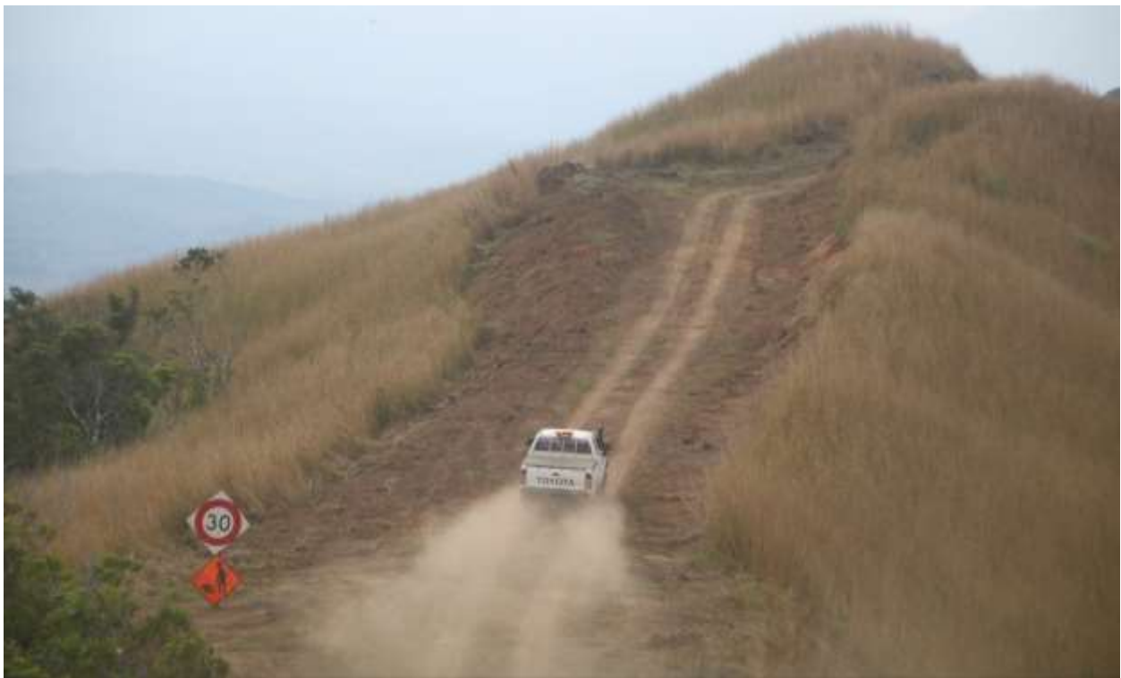
Works in progress on the 14km Matokana Village Access Road by the FRA
