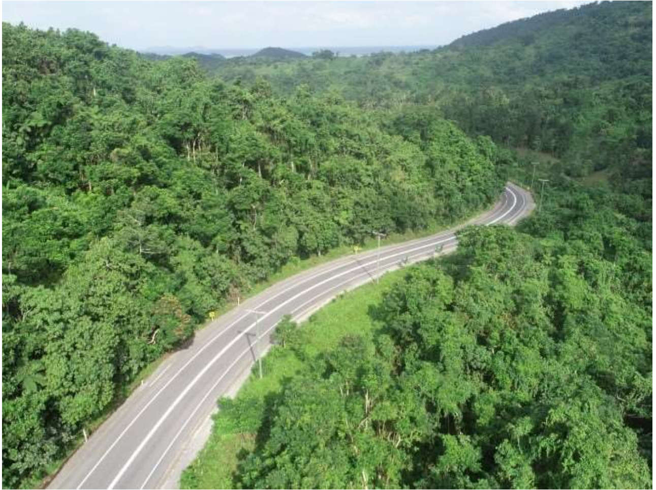
The new and improved Talenaua Section on Queens Road reconstructed by the FRA
