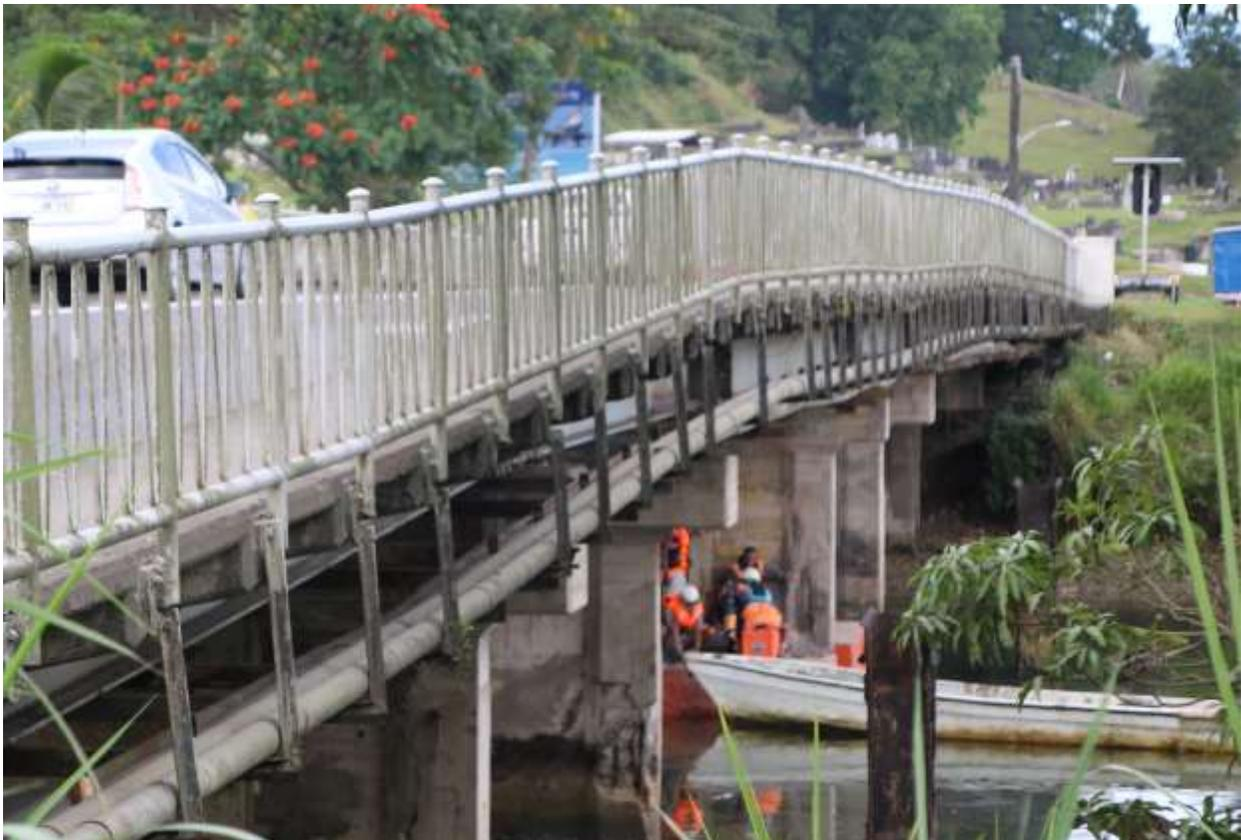
*FRA contractors carrying out maintenance work to the bridge substructure that will provide support to the deck on the Tamavua-i-Wai Bridge on Queens Road.*
