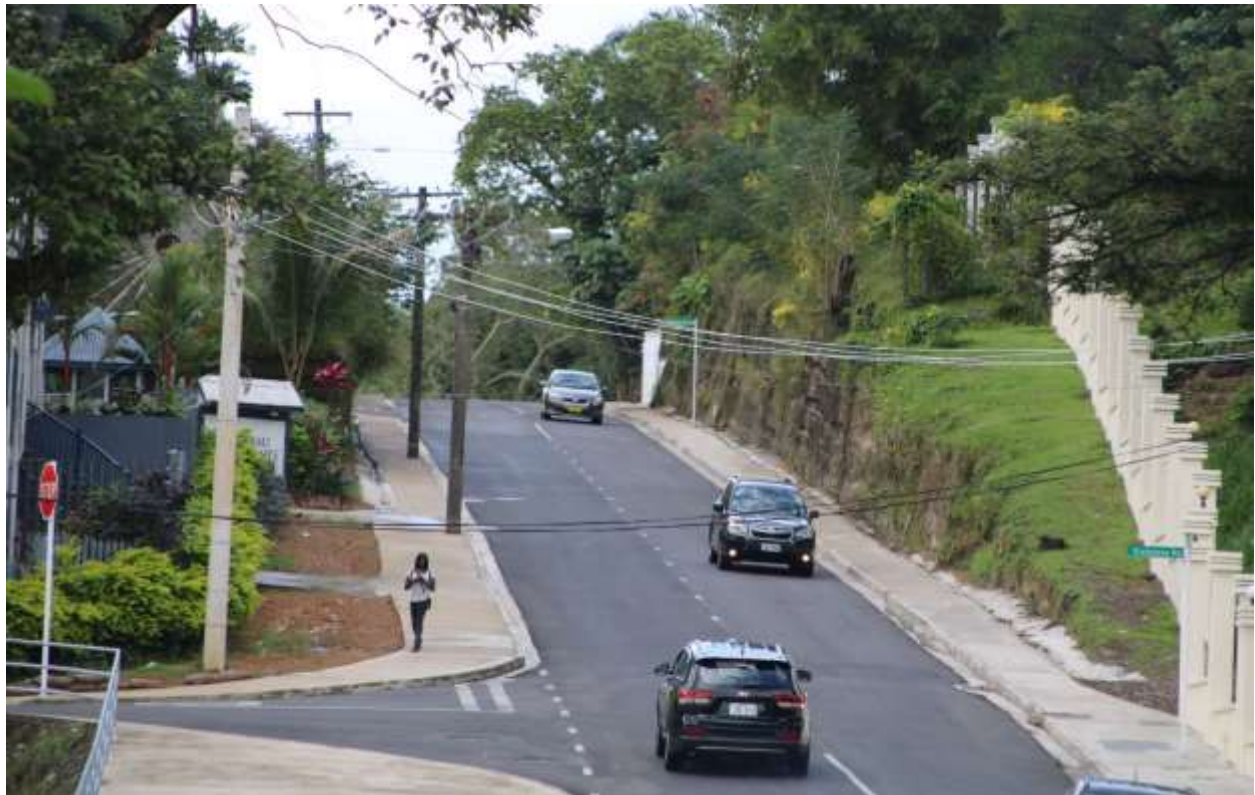
Caption: Rehabilitation works completed at Ratu Cakobau Road in Suva
