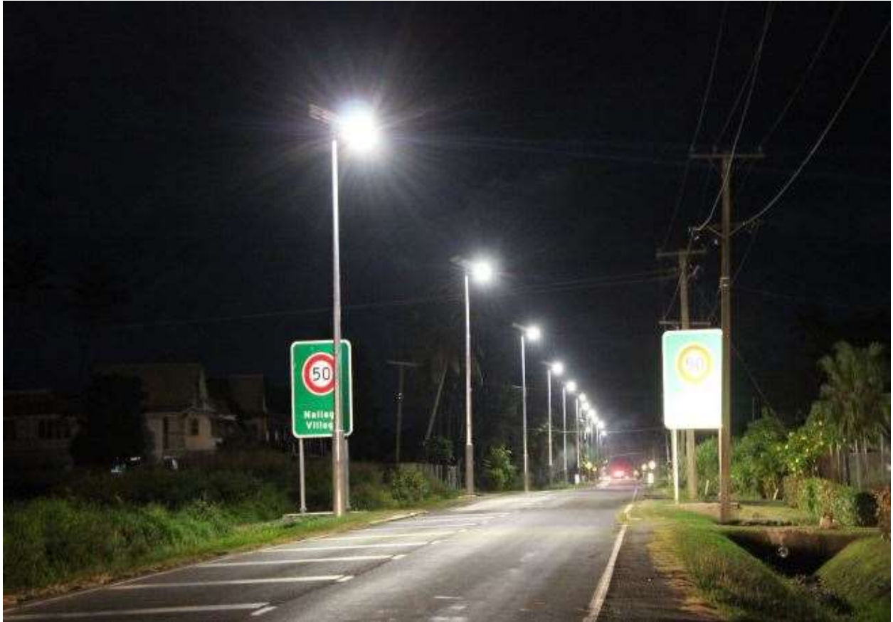
Photo Caption: FRA's first Solar Streetlight Project in Nailaga Village in Ba
