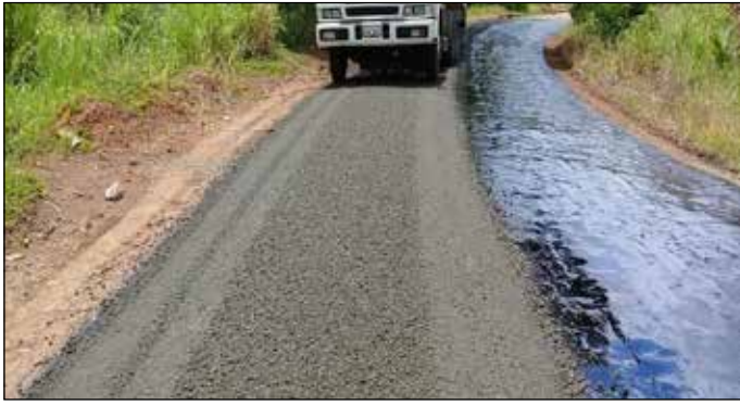
OTTA Surfacing Trial at Bocalevu Road in Labasa
