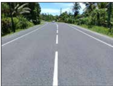
Fiji Roads Authority has successfully completed rehabilitation works on the Naimasimasi Section on Kings Road.
