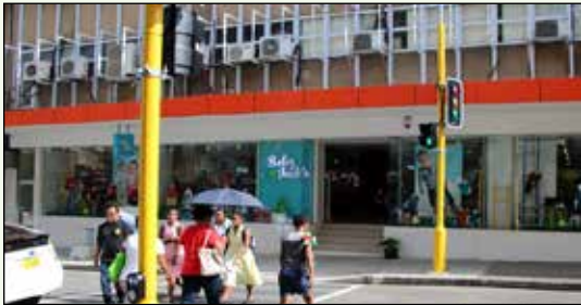
New mid-block pedestrian crossing at Renwick Road
