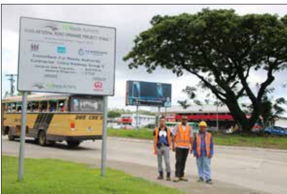
L-R CR5G Site Manager Wang Wan Yin with FRA's SARUP 1 Engineer to Contract Yogesh Raju and CR5G Construction Foreman Chen Chang Lun at the Nabua Roundabout
