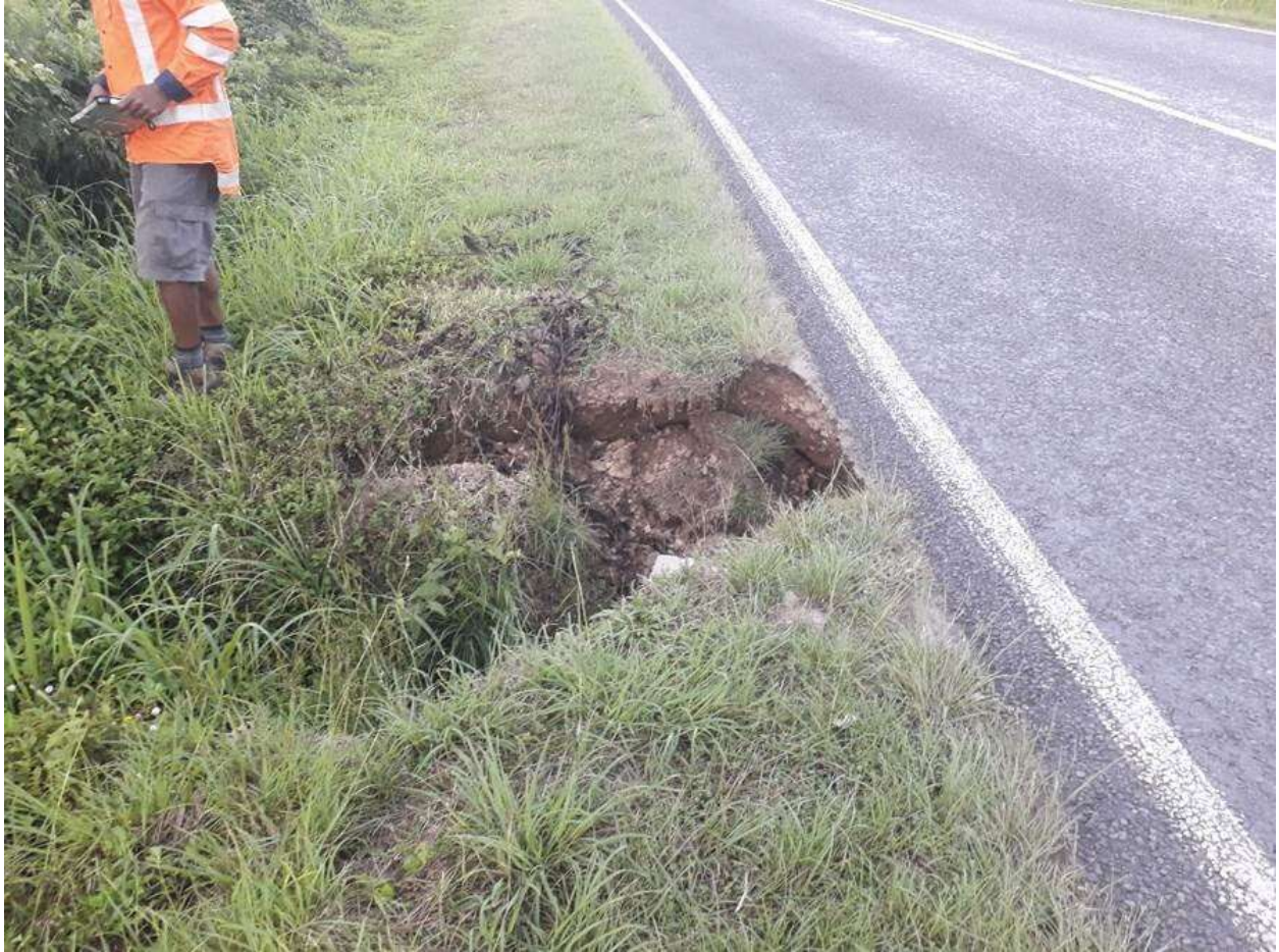
Photo Caption: Drop out on Shoulder of Nadi Bound lane at Bavu Intersection along Queens Road
