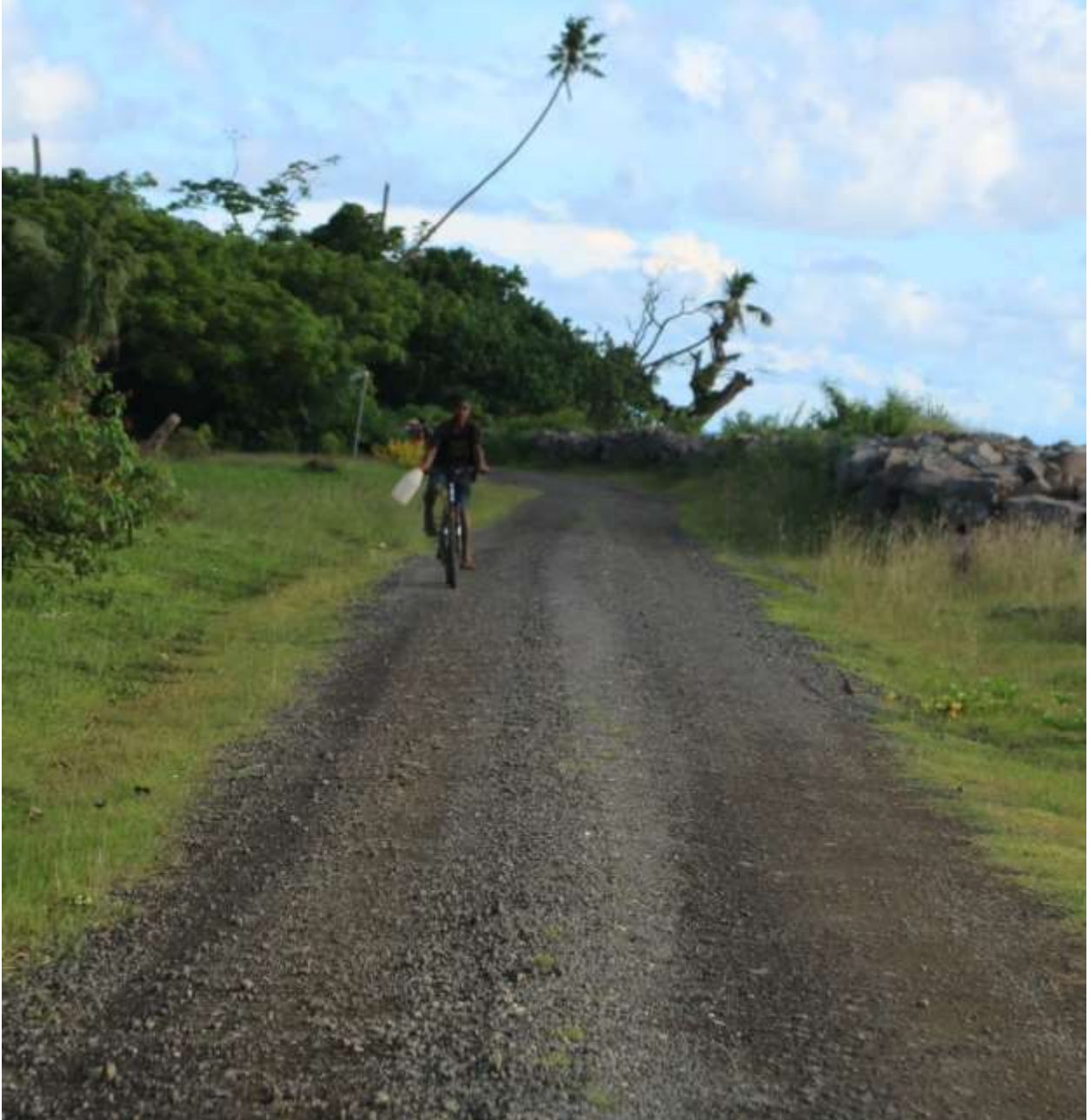
Photo Caption: The new and improved Koro Island Road
