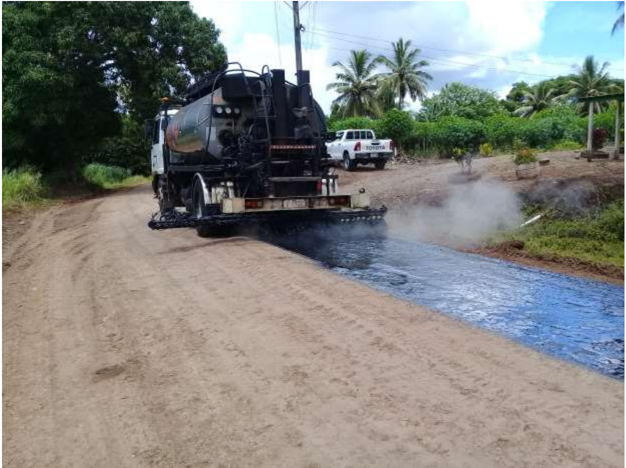
Picture Caption: FRA is trialling OTTA surfacing works at Bocalevu Primary School Frontage on Bocalevu Road in Labasa.
