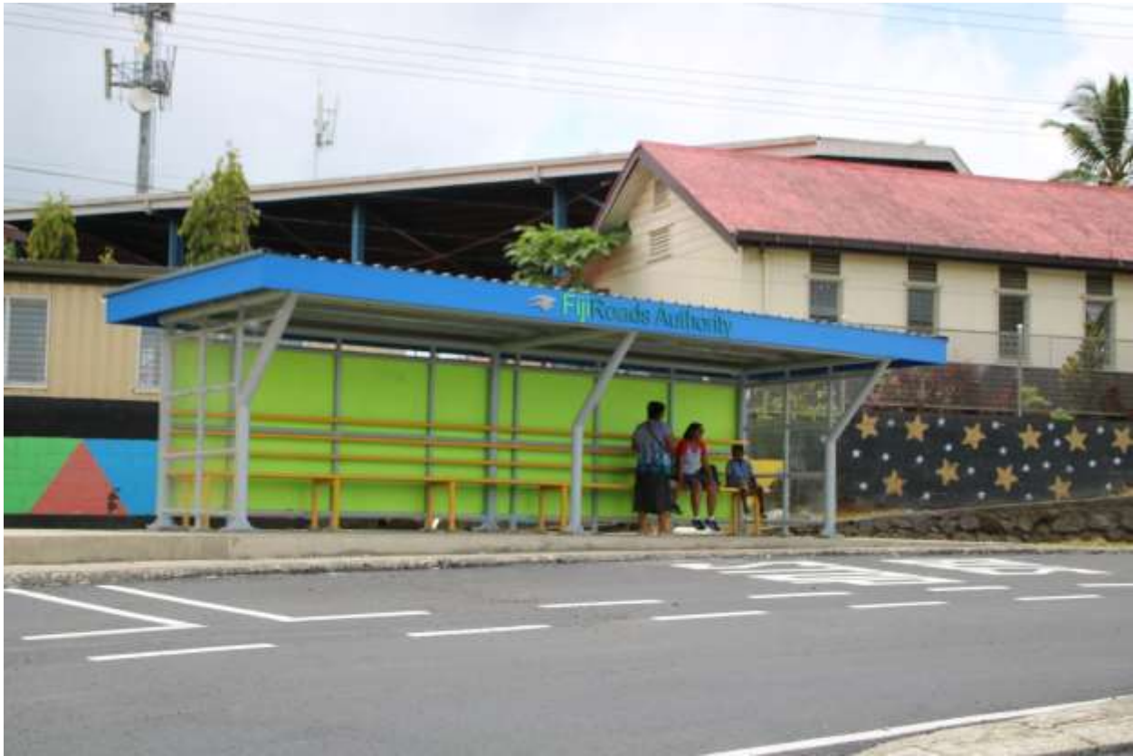
Picture Caption: The new bus shelter in front of Tamavua Primary School constructed by the FRA
